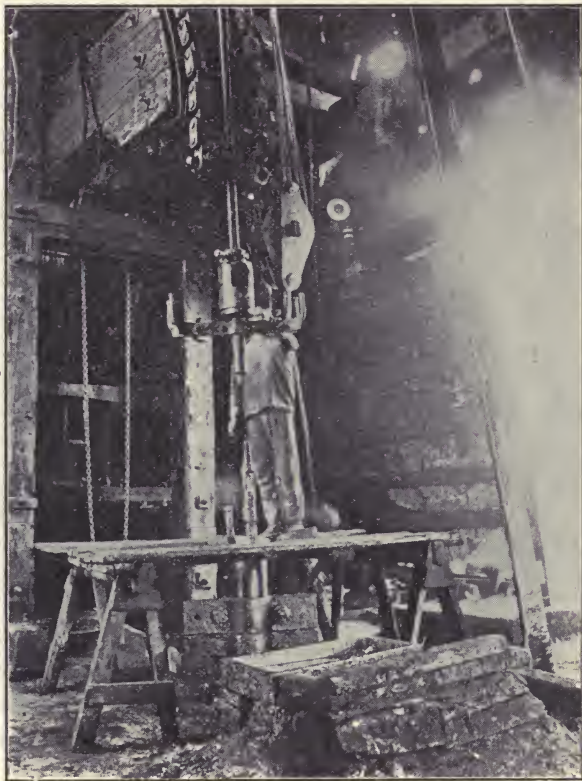
FIG. 3.—INTERIOR OF DERRICK SHOWING END OF WALKING BEAM AND TEMPER-SCREW
