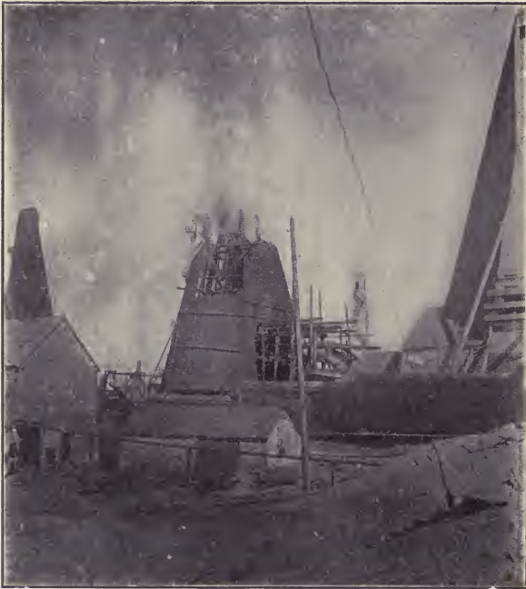
FIG. 4.—WELL BLOWING OUT THROUGH 26-IN. CASING. MAKING GAS, WATER AND LARGE QUANTITIES OF SAND.
