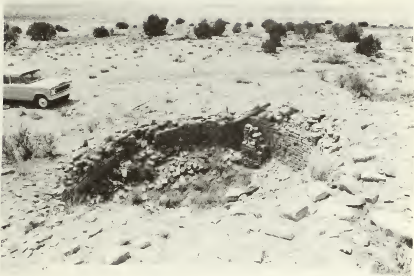
Kiva, west wall: before stabilization
