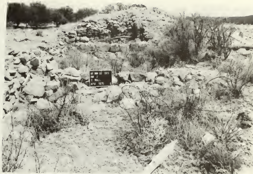
Room 2, east wall: before stabilization
