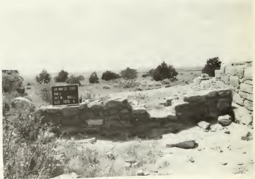
Room 3, west wall: after stabilization
