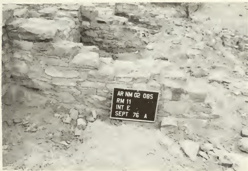
Room 11, east wall: after stabilization
