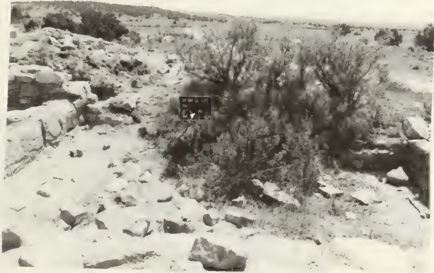
Room 3, south wall: after stabilization
