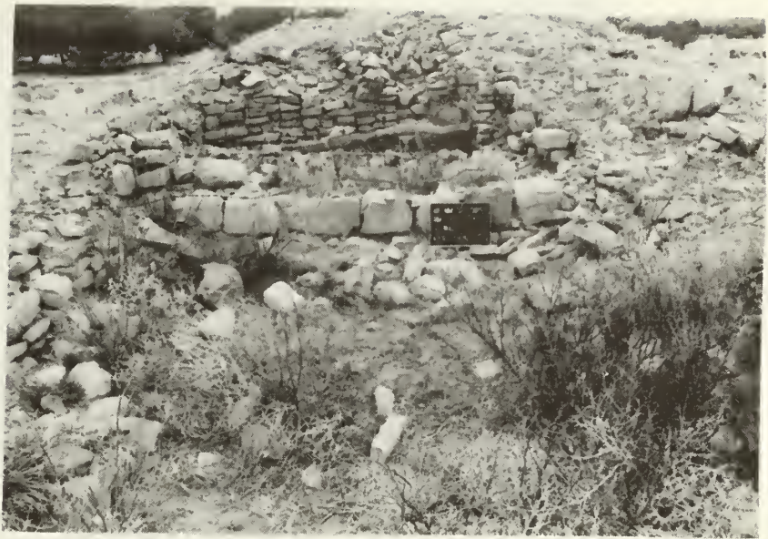
Room 3, east wall: before stabilization
