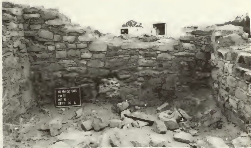
Room 10, north wall: after stabilization
