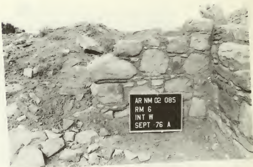
Room 6, west wall: after stabilization
