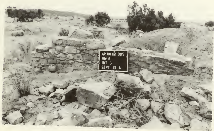
Room 8, south wall: after stabilization
