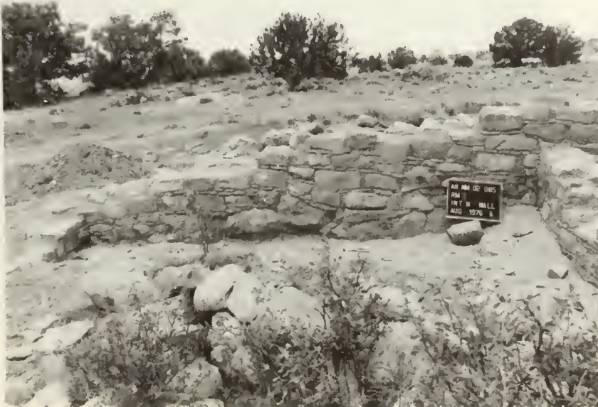
Room 2, north wall: after stabilization
