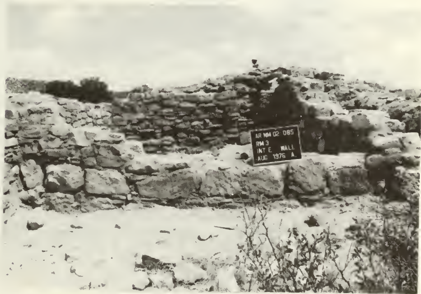
Room 3, east wall: after stabilization
