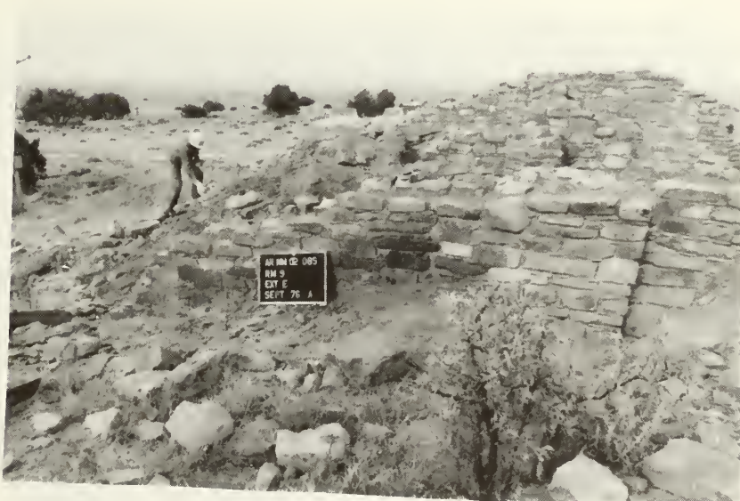
Room 9, exterior of east wall: after stabilization
