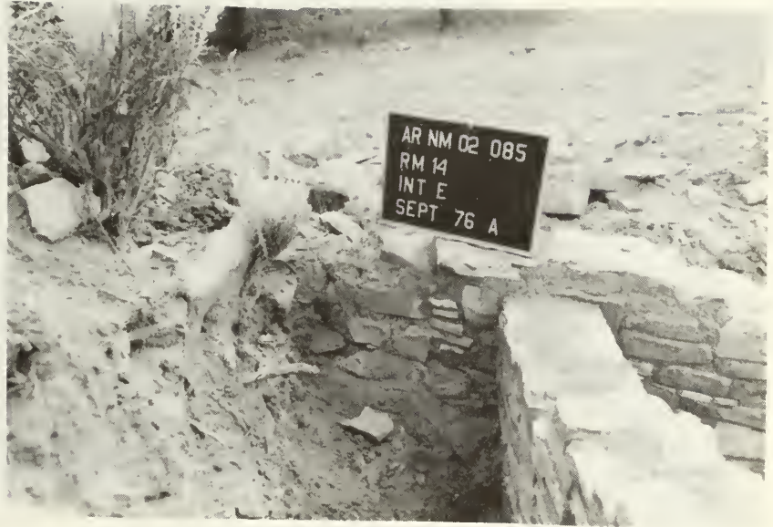
Room 14, east wall: after stabilization
