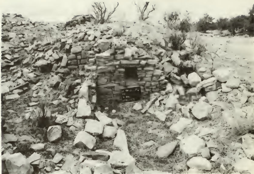
Room 7, north wall: before stabilization
