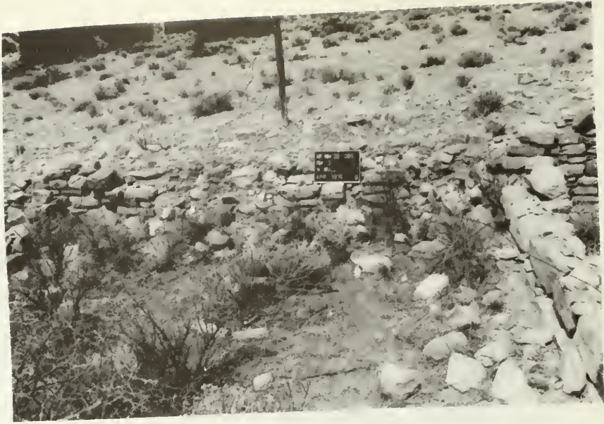
Room 3, north wall: before stabilization
