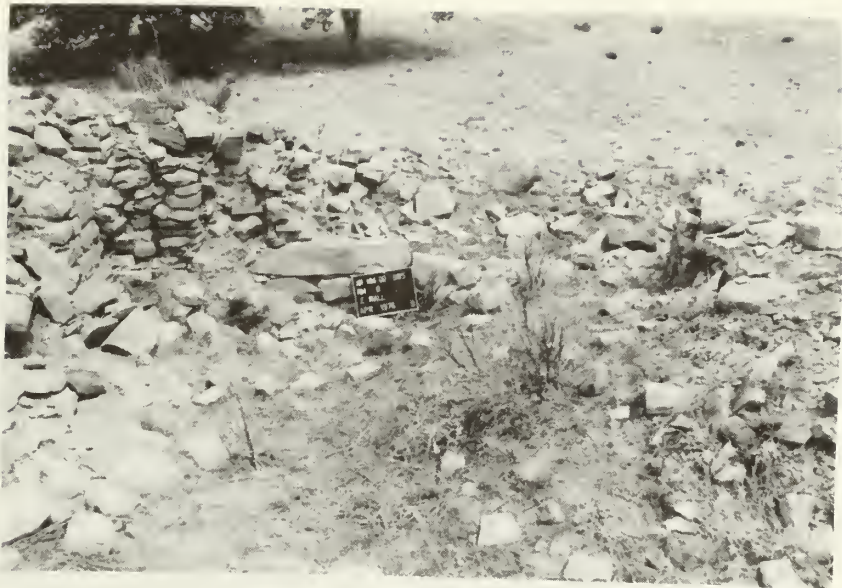
Room 8, east wall: before stabilization
