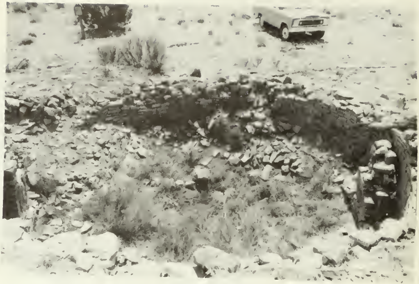
Kiva, south wall: before stabilization
