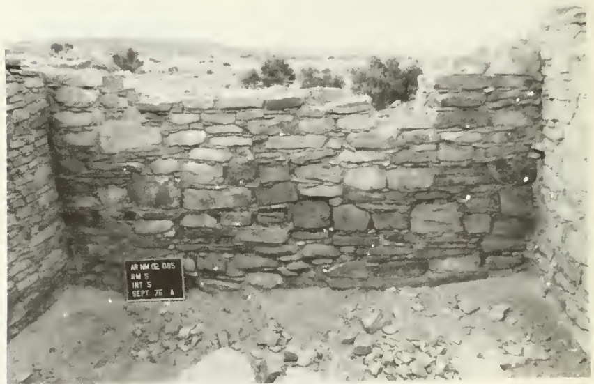
Room 5, south wall: after stabilization
