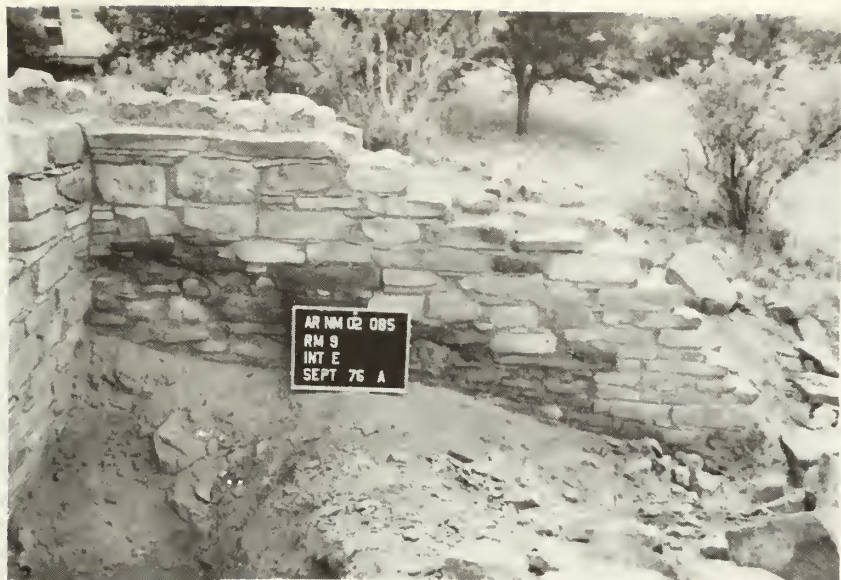
Room 9, east wall: after stabilization
