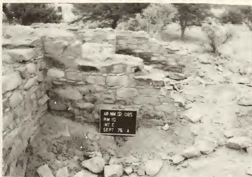
Room 10, east wall: after stabilization
