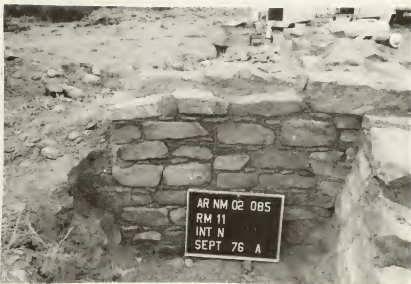
Room 11, north wall, after stabilization
