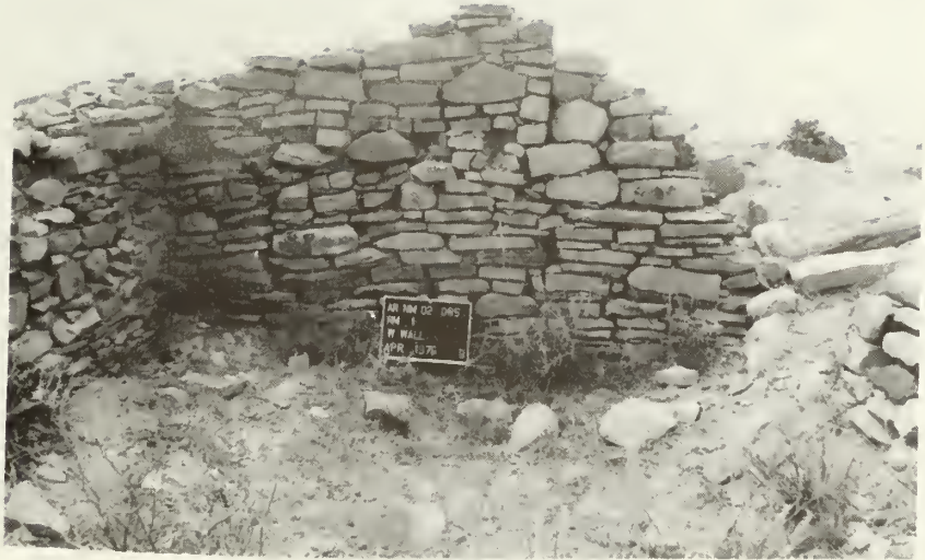
Room 1, west wall: before stabilization
