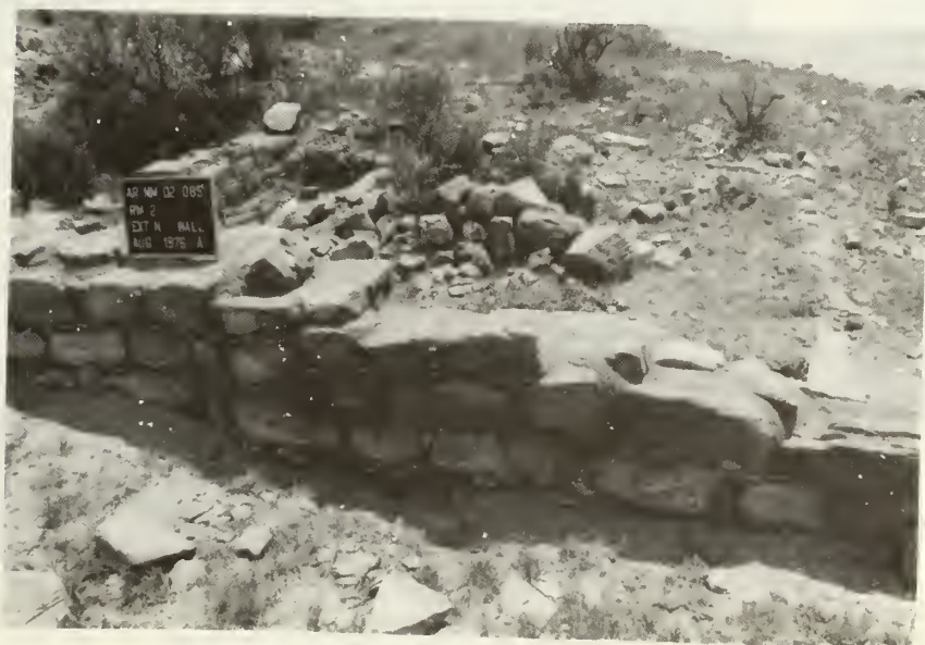
Room 2, north wall: after stabilization
