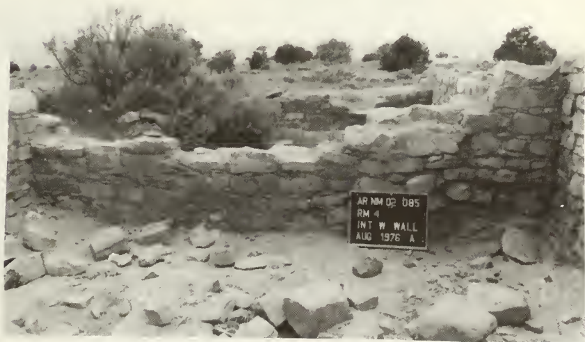
Room 4, west wall: after stabilization
