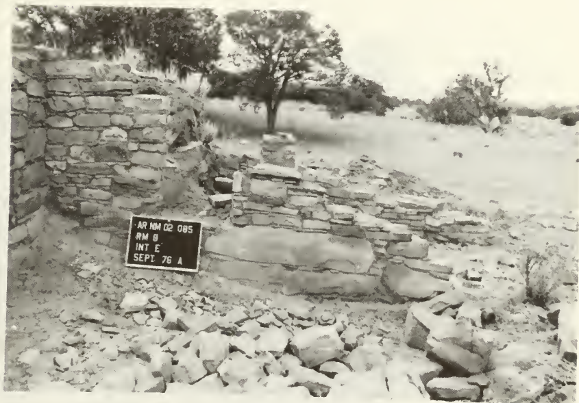
Room 8, east wall: after stabilization
