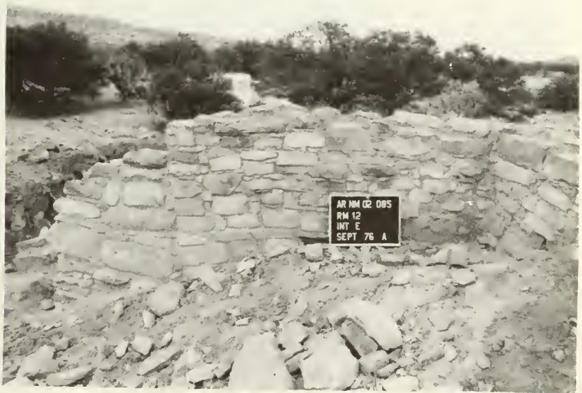
Room 12, east wall: after stabilization
