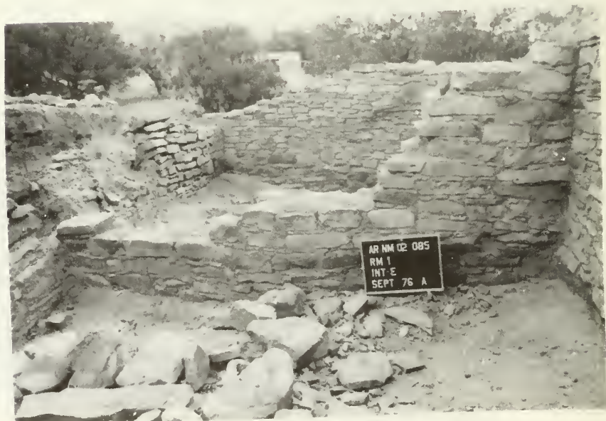
Room 1, east wall: after stabilization
