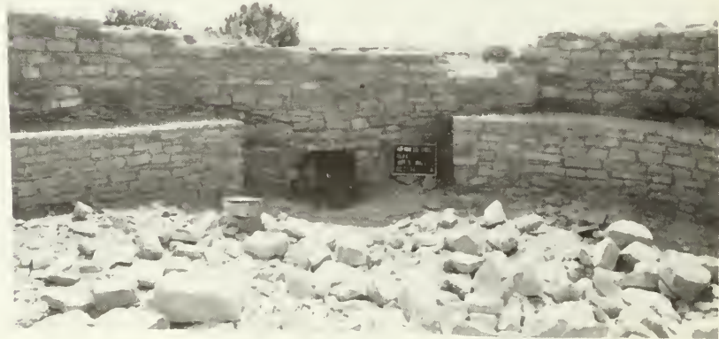
Kiva, south wall: after stabilization
