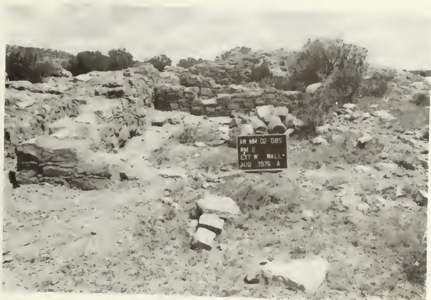
Room 2, west wall: after stabilization
