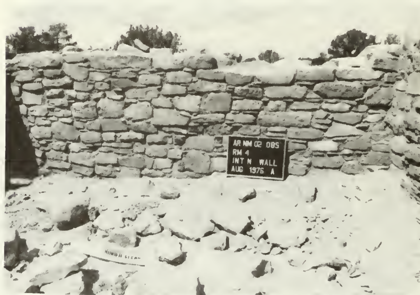
Room 4, north wall: after stabilization
