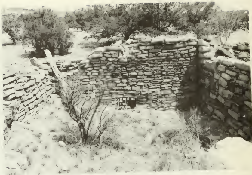
Room 5, east wall: before stabilization
