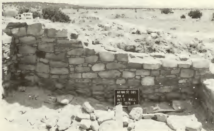
Room 4, south wall: after stabilization
