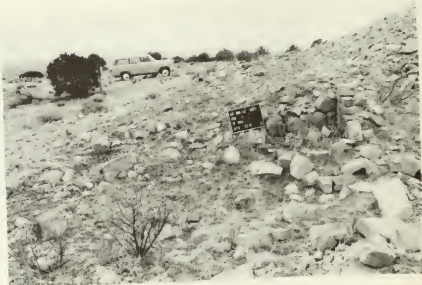
Room 6, west wall: before stabilization
