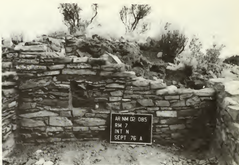
Room 7, north wall: after stabilization
