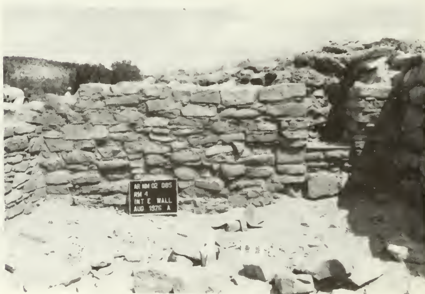
Room 4, east wall: after stabilization.
