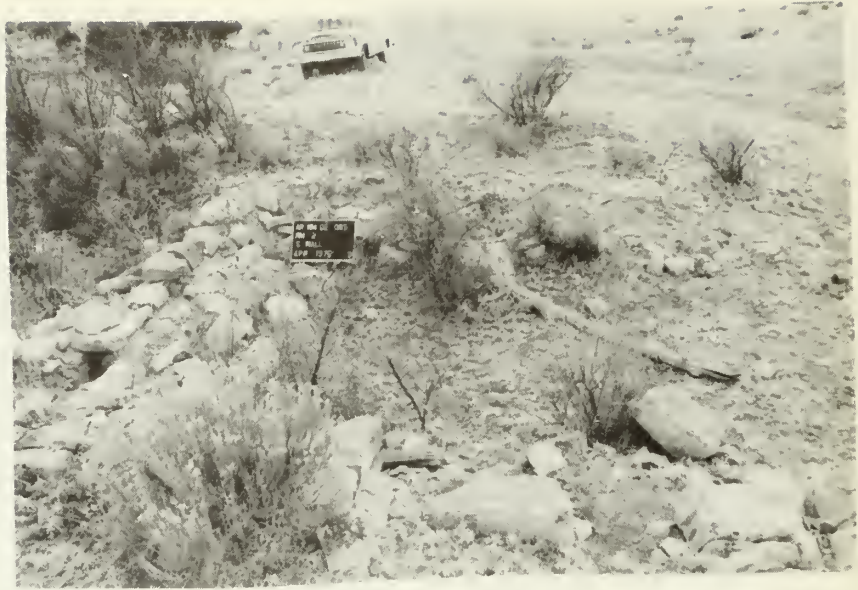
Room 2, south wall: before stabilization
