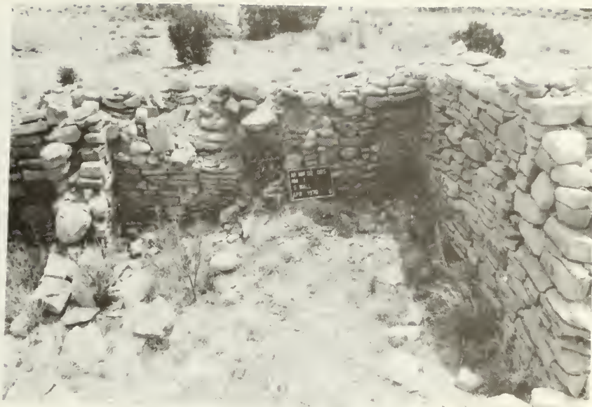
Room 1, south wall: before stabilization
