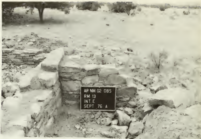
Room 13, east wall: after stabilization
