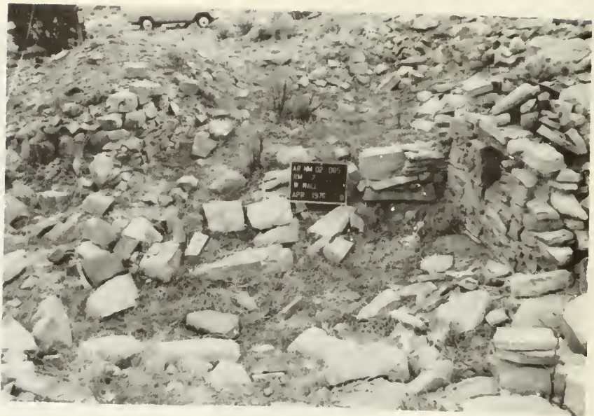
Room 7, west wall: before stabilization
