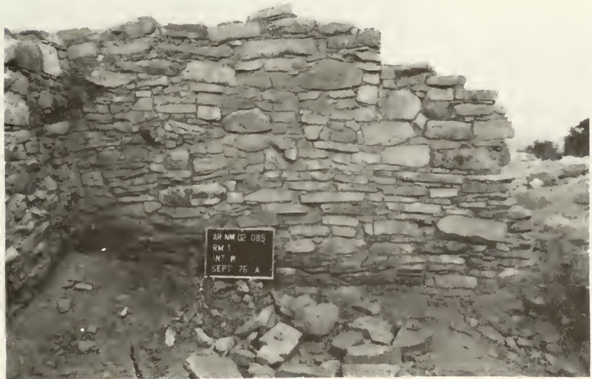
Room 1, west wall: after stabilization
