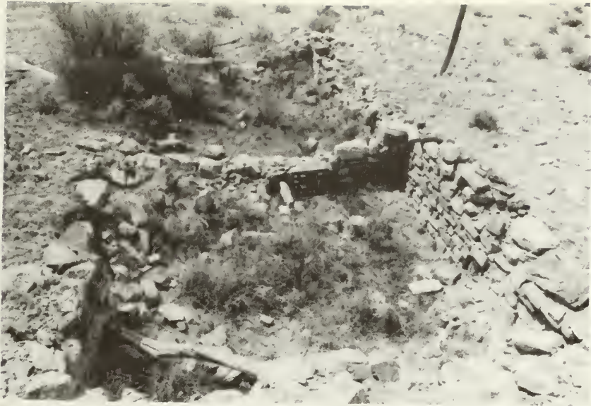
Room 4, west wall: before stabilization
