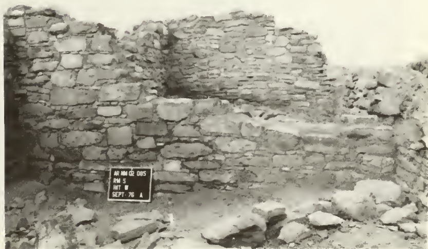
Room 5, west wall: after stabilization
