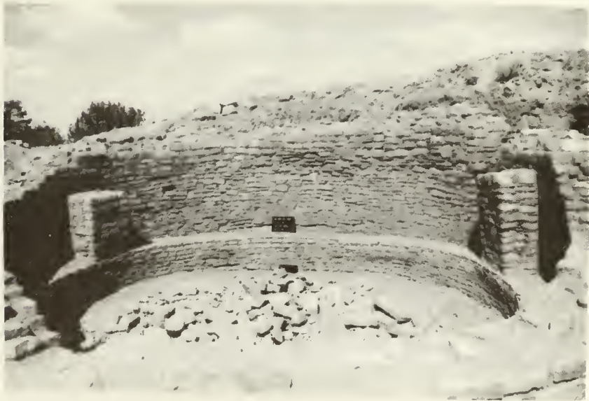
Kiva, north wall: after stabilization
