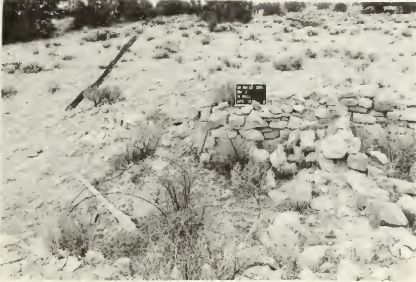
Room 2, north wall: before stabilization
