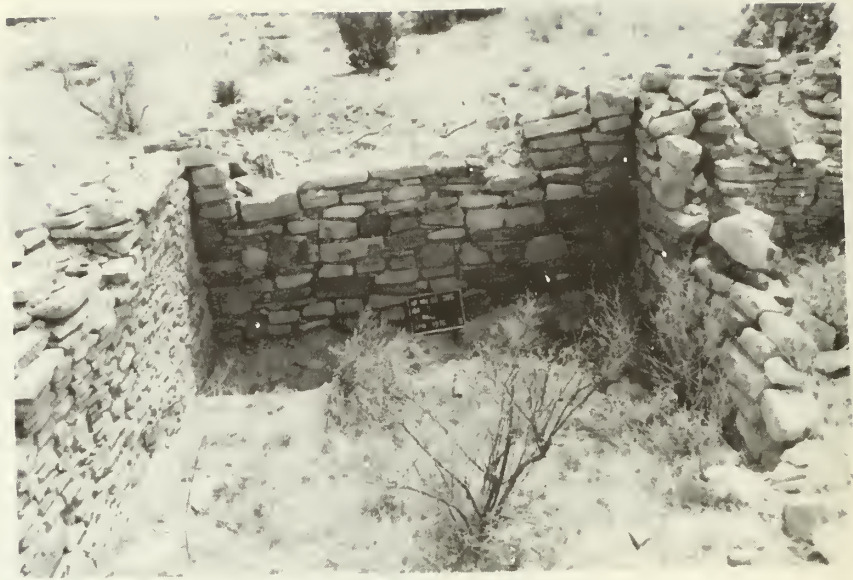
Room 5, south wall: before stabilization
