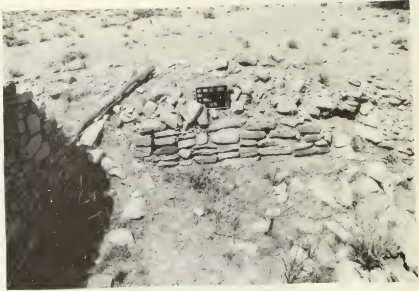
Room 1, north wall: before stabilization
