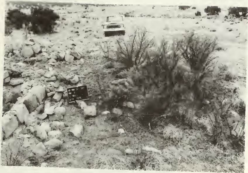
Room 3, south wall: before stabilization
