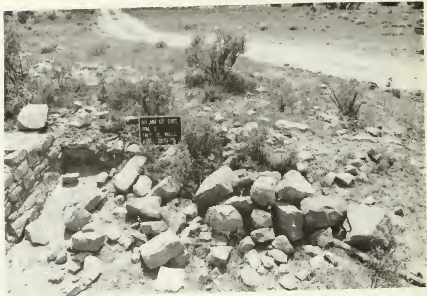
Room 2, south wall: after stabilization
