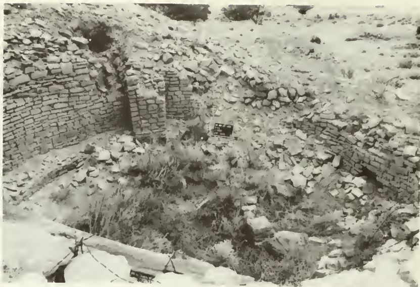
Kiva, east wall: before stabilization
