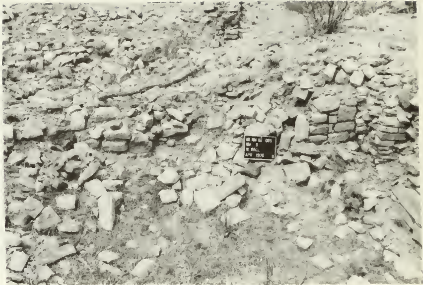
Room 8, north wall: before stabilization
