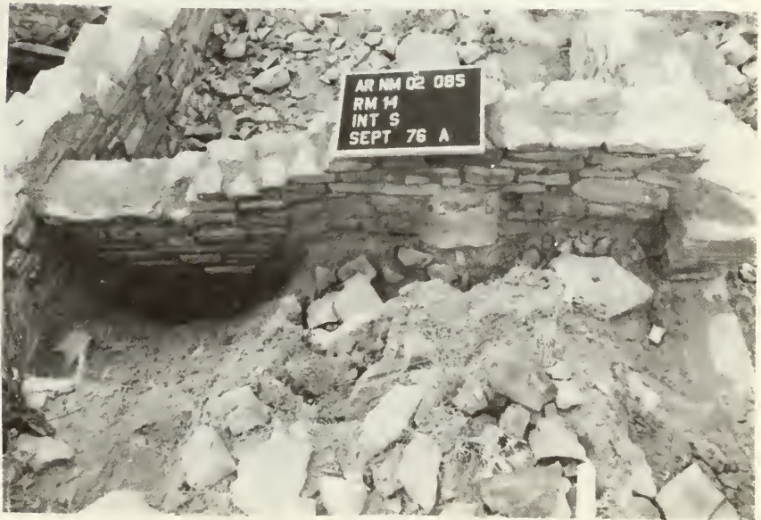
Room 14, south wall: after stabilization
