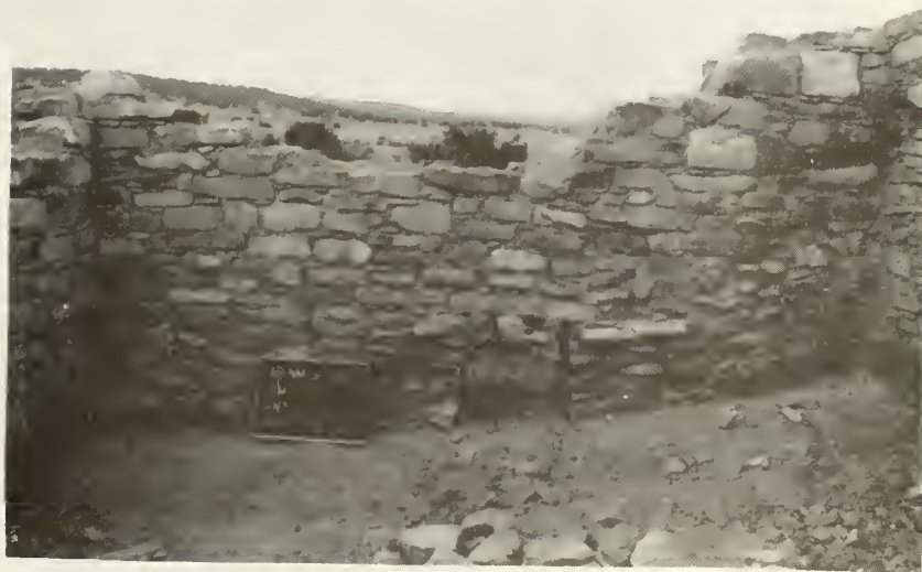
Room 1, south wall: after stabilization
