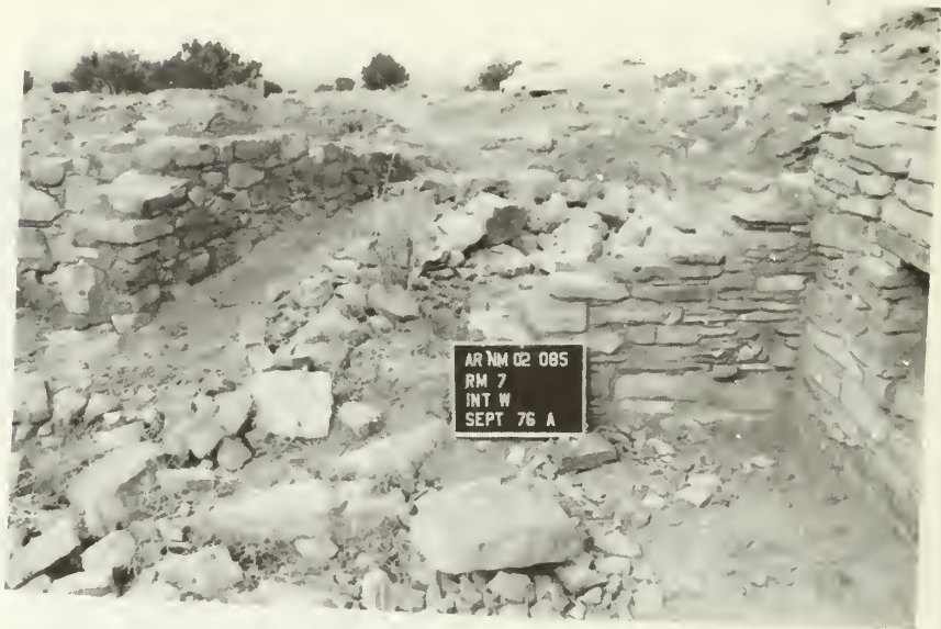
Room 7, west wall: after stabilization
