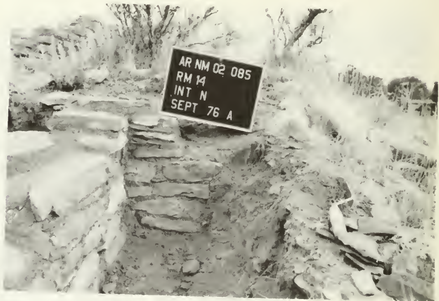
Room 14, north wall: after stabilization
