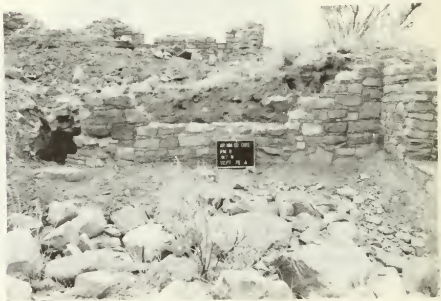
Room 8, north wall: after stabilization
