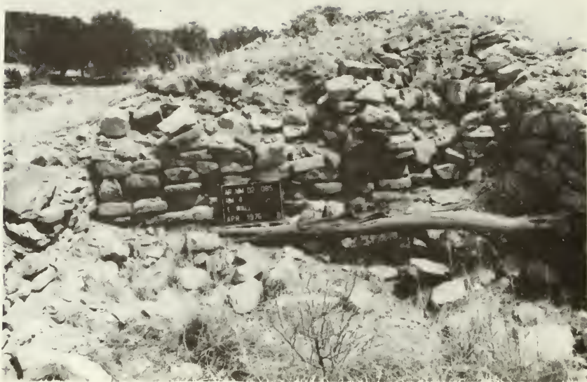
Room 4, east wall: before stabilization
