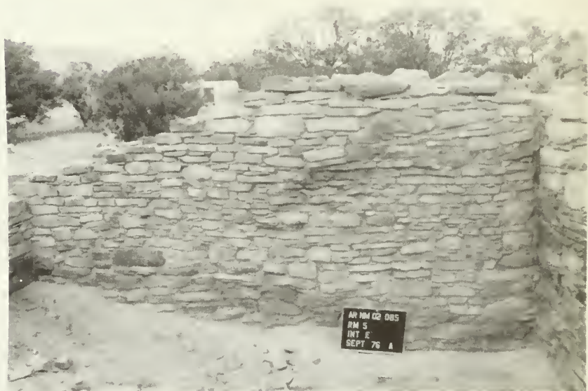
Room 5, east wall: after stabilization
