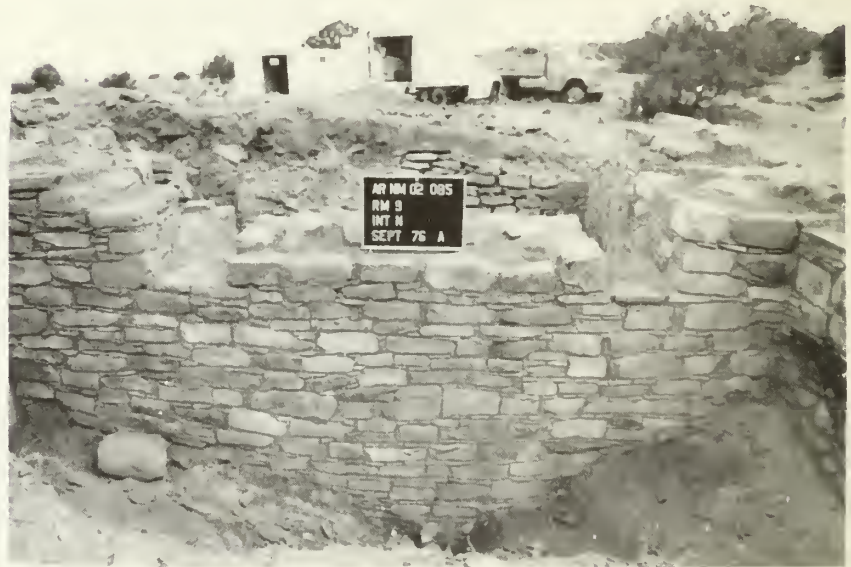
Room 9, north wall: after stabilization
