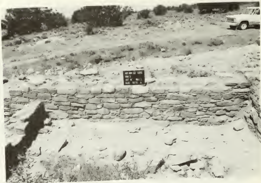
Room 3, north wall: after stabilization
