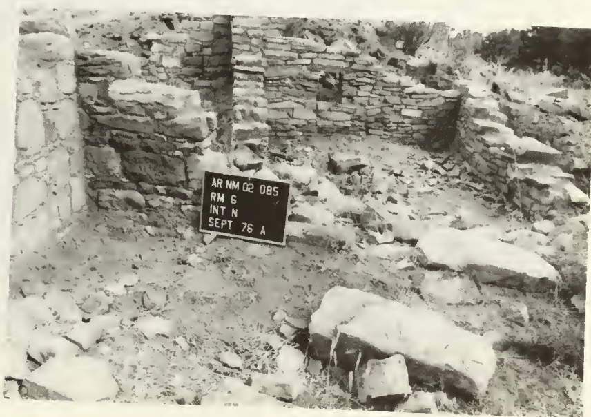
Room 6, north wall: after stabilization
