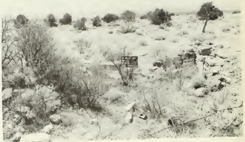
Room 3, west wall: before stabilization
