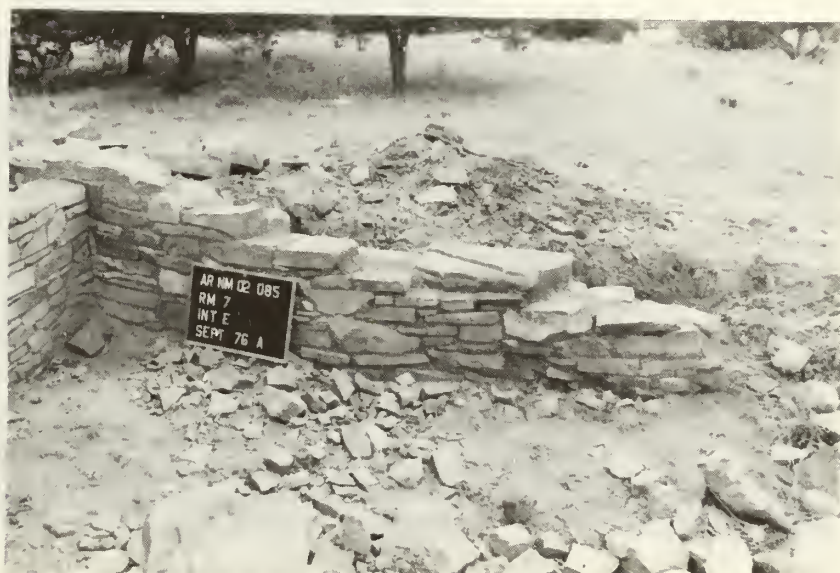
Room 7, east wall: after stabilization
