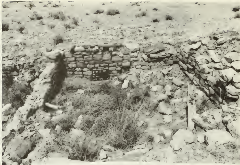
Room 4, north wall: before stabilization
