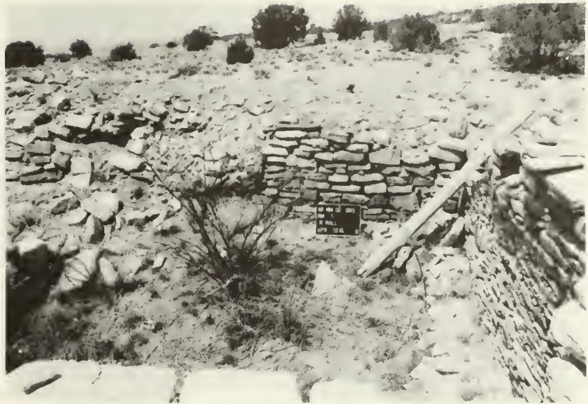
Room 5, north wall: before stabilization
