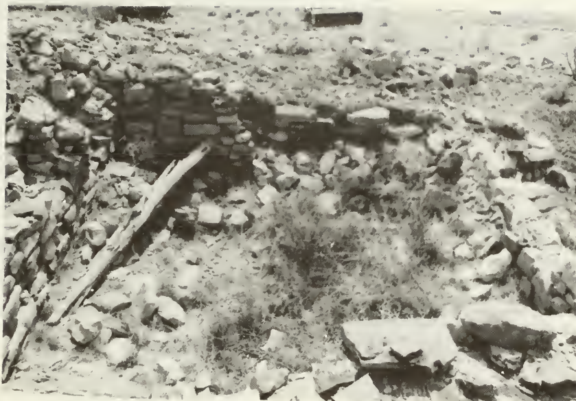
Room 4, south wall: before stabilization
