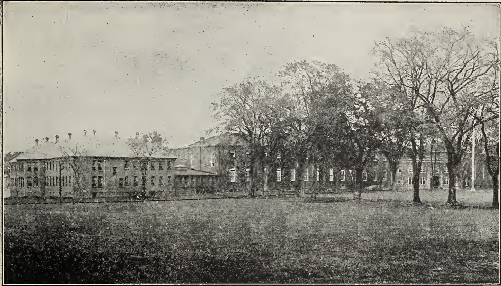
CONNECTICUT STATE PRISON—Situated at Wethersfield.
