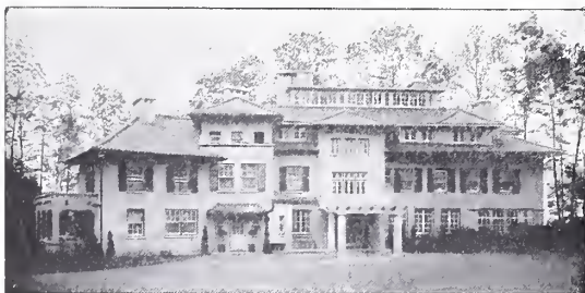
Residence of Wm. C. DeLaney, Esq., Short Hills, N. J. John A. Gard, Architect Reinforced Concrete throughout. Roof, Green Tile laid on Reinforced Concrete
