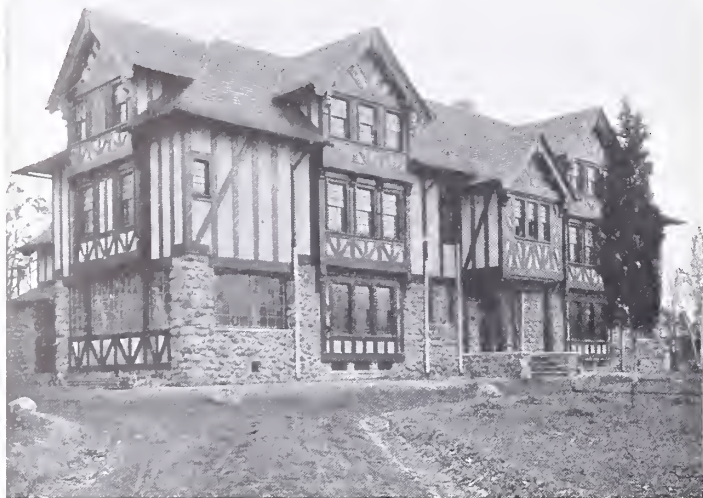
SUBURBAN RESIDENCE OF WM. DORFLINGER, ESSEX FELLS, N. J. Lighted by 100-Light Sunlight "Omega" Generator
