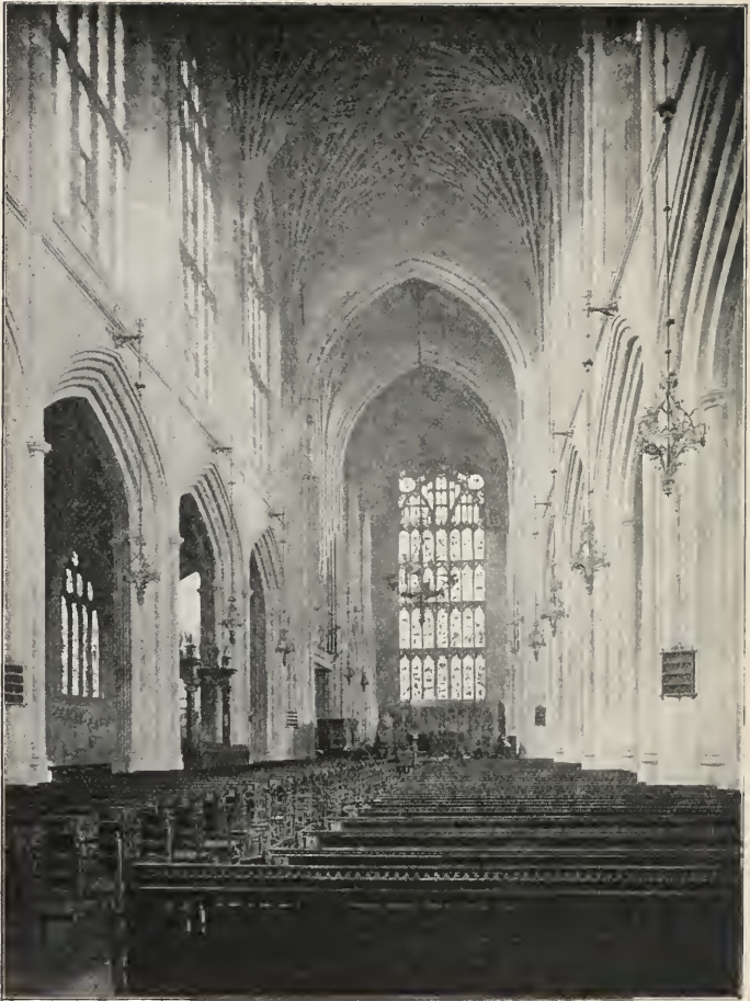
THE NAVE, LOOKING EAST.
