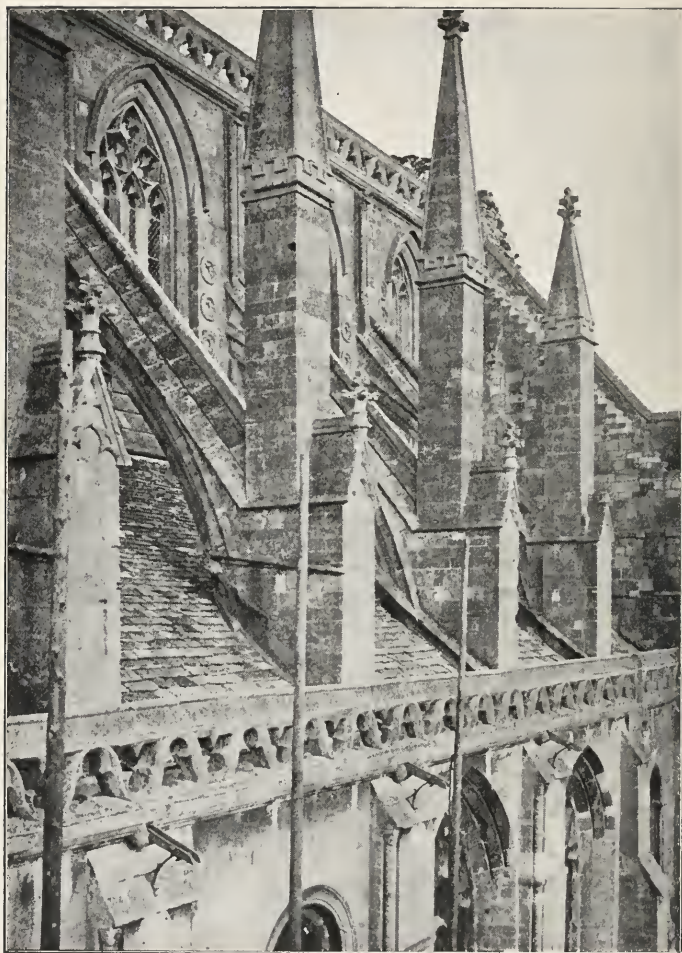
THE SOUTH SIDE FROM THE PORCH ROOF.
