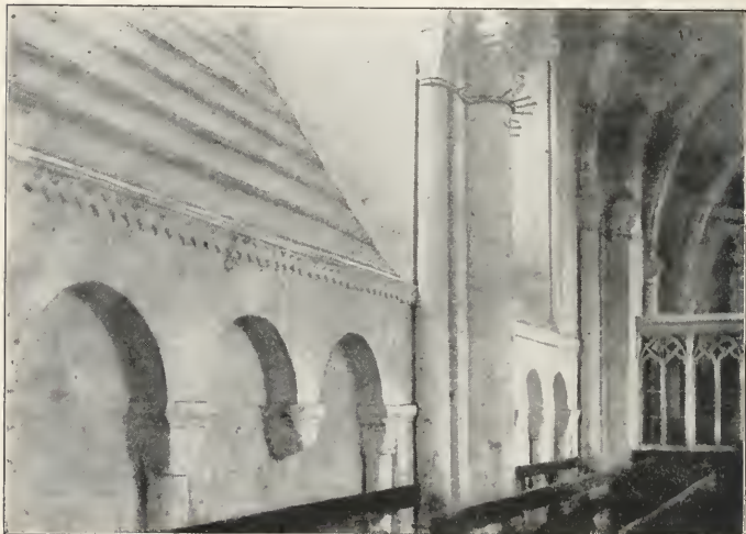
WALL ARCADE, NORTH SIDE.
