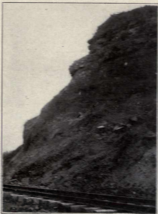
24. ESTILL SHALE UNDERLYING COLUMBUS LIMESTONE Winchester-Irvine Branch of the Louisville and Nashville Railroad, Estill County. Photograph by A. M. Miller
