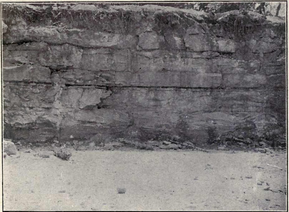
17. EXPOSURE OF WAYNESVILLE LIMESTONE
