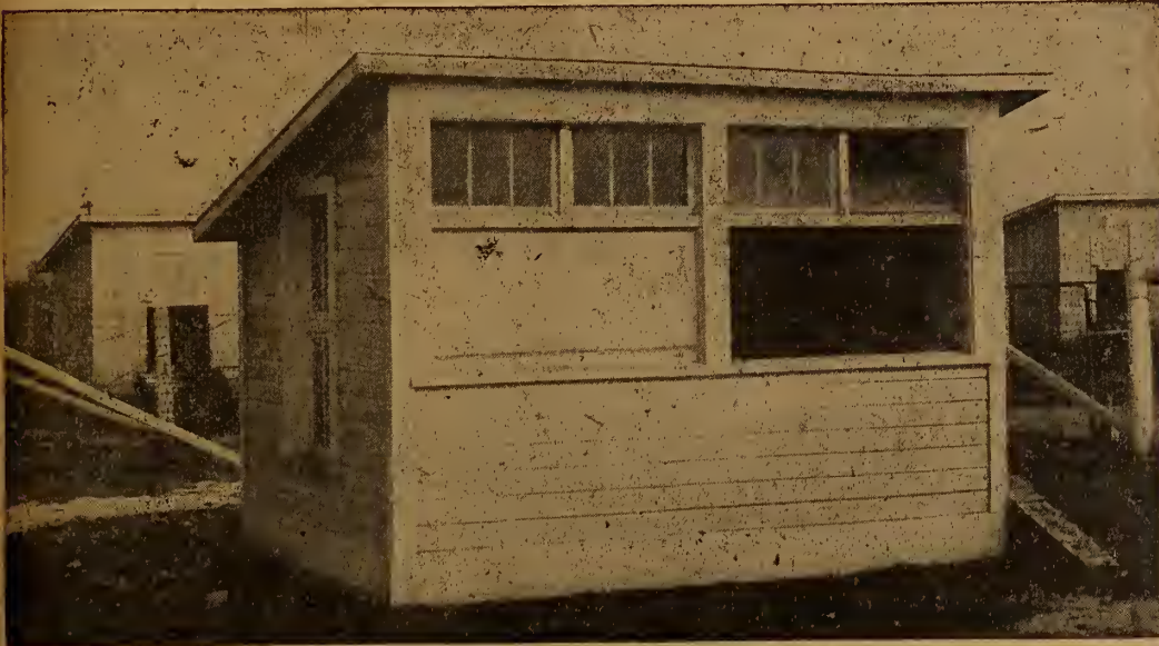
A small open-front, fresh air breeding house, well suited for the Southern climate.
