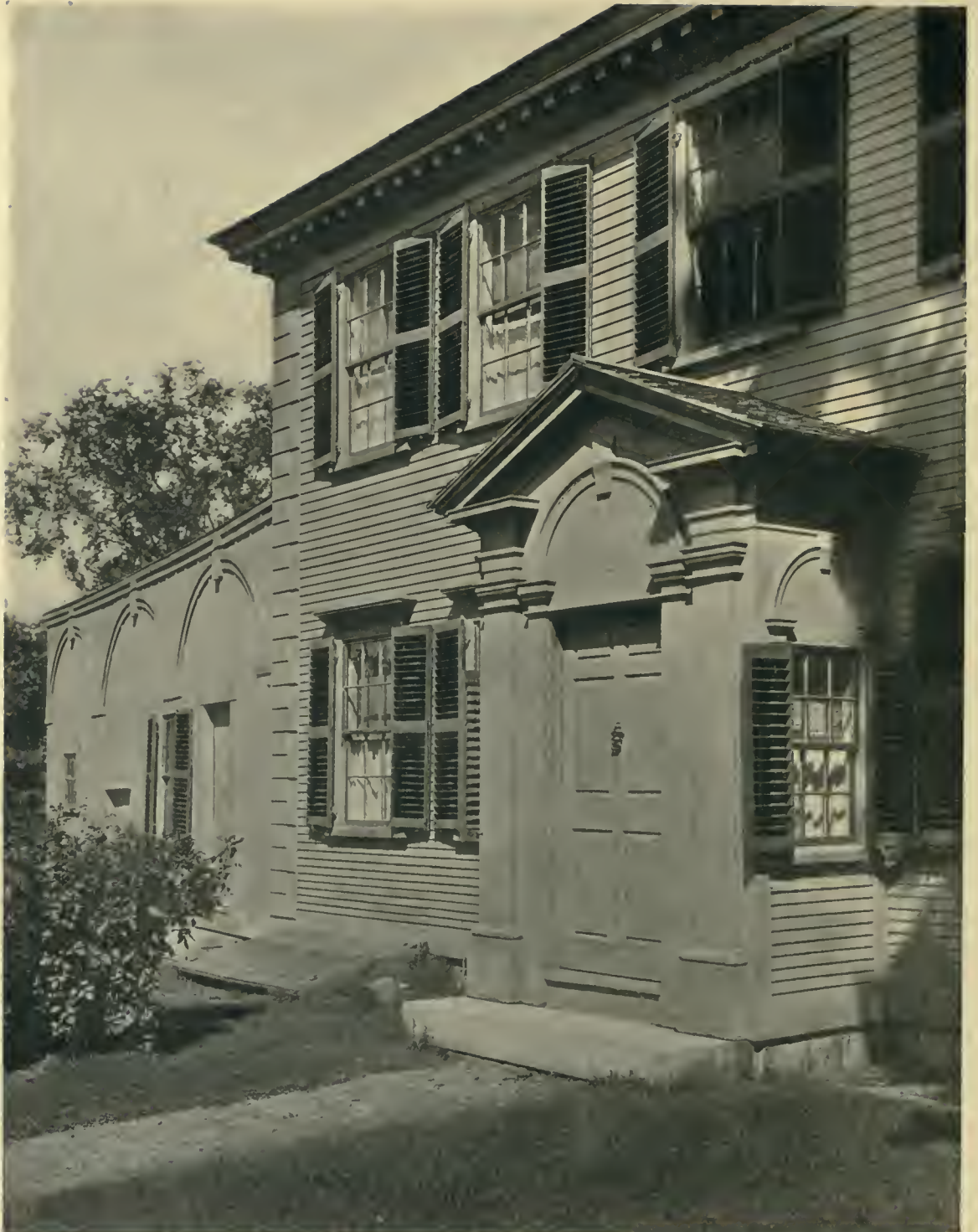
THE OLD SWIFT HOUSE, ANDOVER, MASSACHUSETTS. Built in 1795. Detail of Side Doorway and Vestibule.
