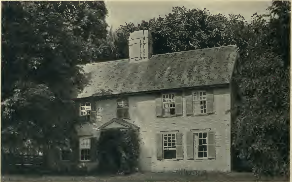
"GOVERNOR BRADSTREET HOUSE," NORTH ANDOVER, MASSACHUSETTS.
