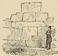
Fig. 109. WALL AT FIESOLE.
