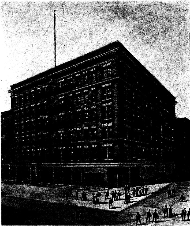
Built by A. B. KIGHT 1907-8
