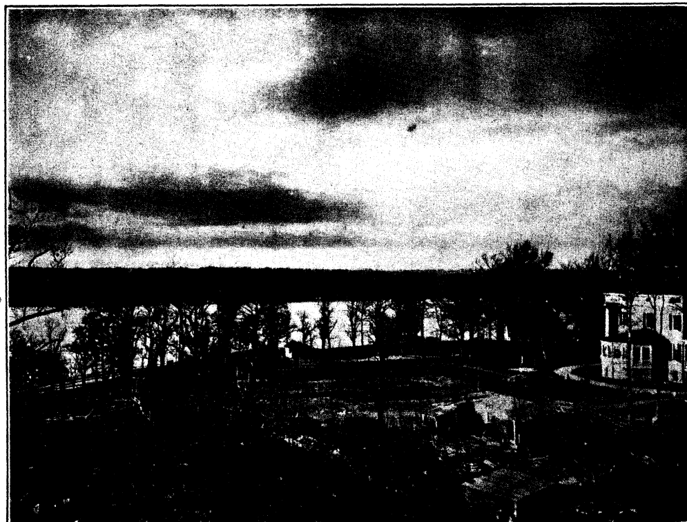
VIEW LOOKING NORTH
