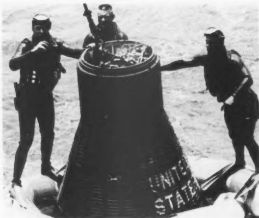
Navy frogmen attach flotation ring to Faith Seven prior to its recovery by USS Kearsarge near Midway.
