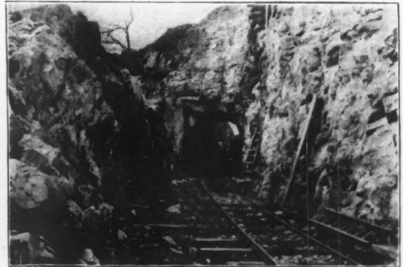
FIG. 3.—TUNNEL AND ROCK CUT AT POLNISH.
