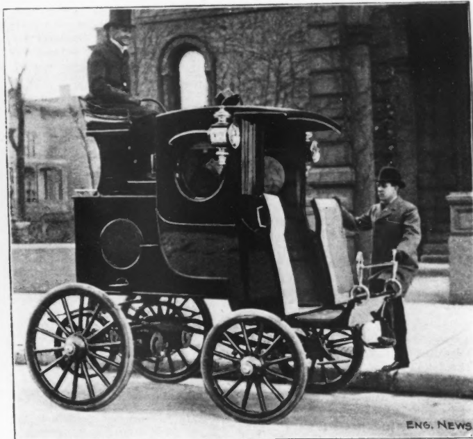
FIG. 2.—HANSOM CAB OPERATED BY STORAGE BATTERIES. FISCHER EQUIPMENT CO., MAKERS.
