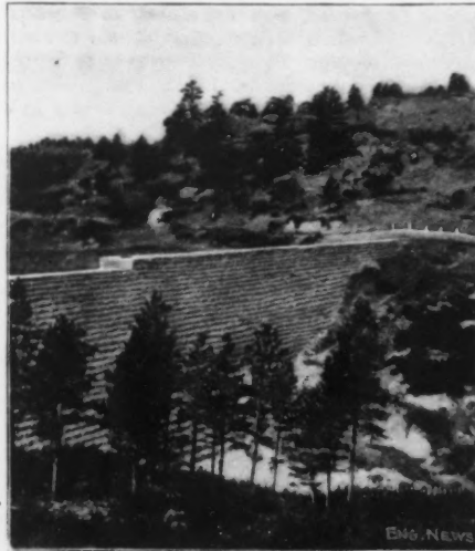
Fig. 3.—View of Castlewood Dam from Below.
