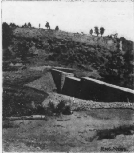
Fig. 2.—View of Castlewood Dam from Above Showing Earth Embankment, Riprapped.
