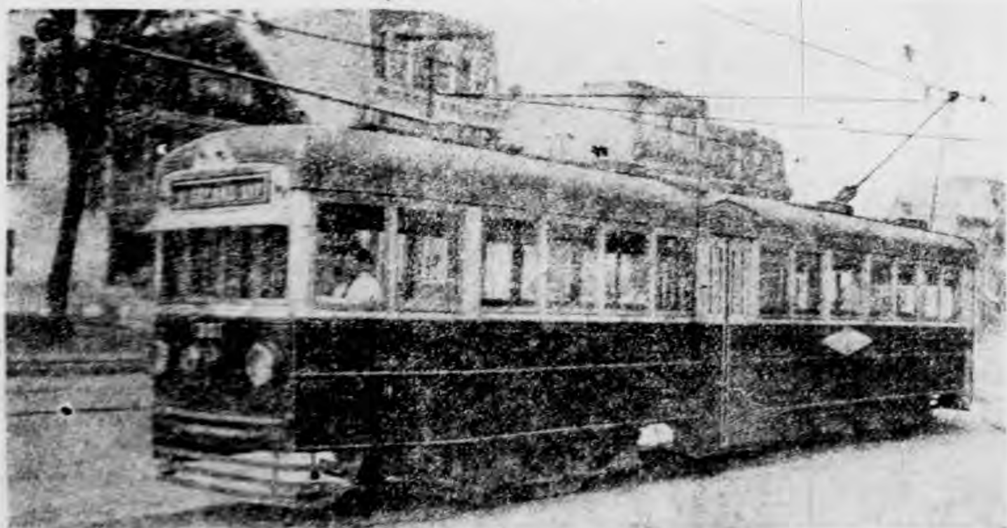
Fig 27. Light-weight Car with Electro-pneumatic Control; United Traction Company, Albany (N. Y.)
