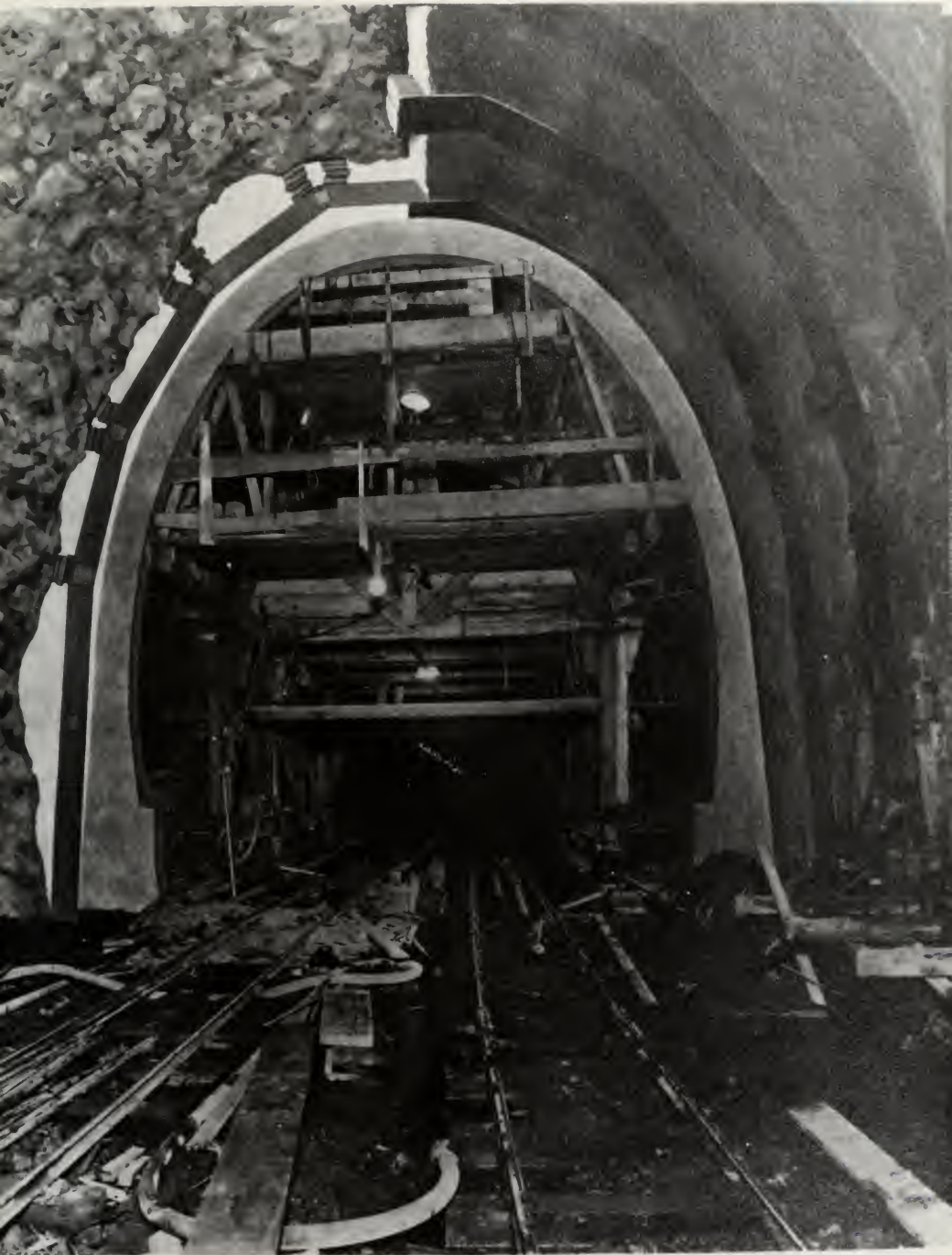
SCHEMATIC PHOTOGRAPH SHOWING CROSS-SECTION OF LINING. TYPE "I" METHOD.
