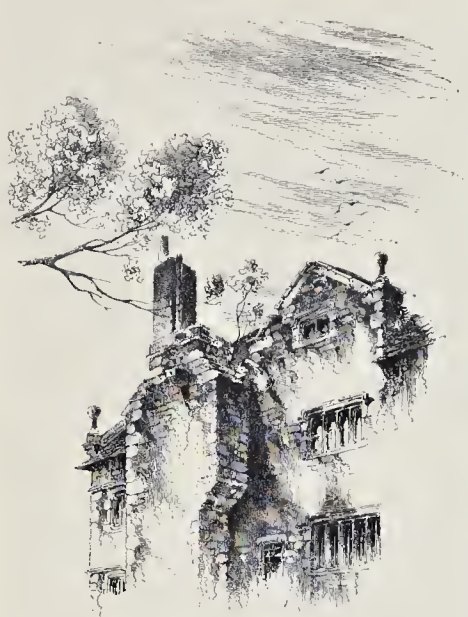
No. 4.—A Chimney, East Front, Livesey Hall.
