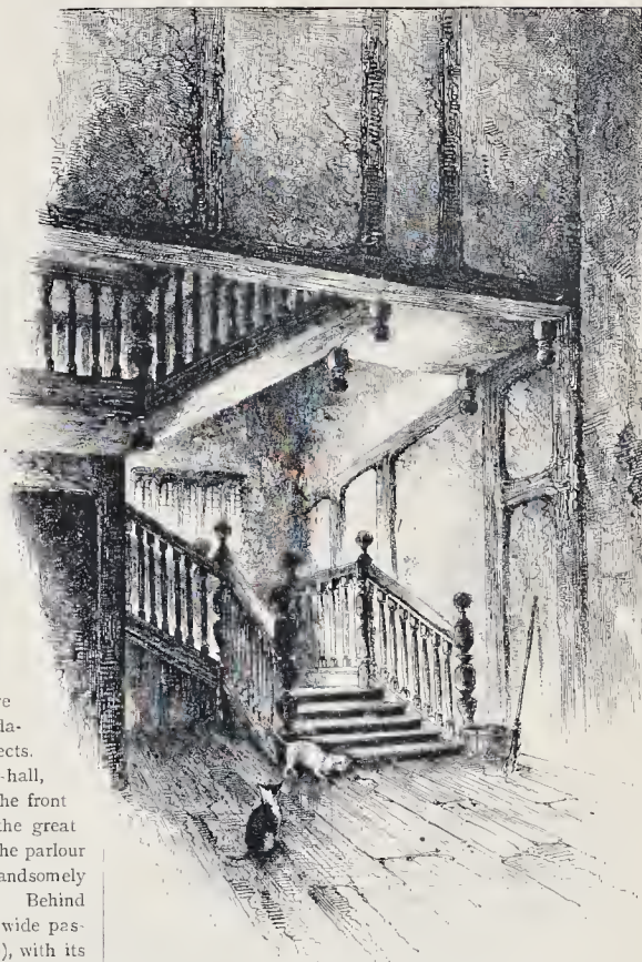
No. 6.—The Staircase, Livesey Hall. Drawn by H. Railton.
