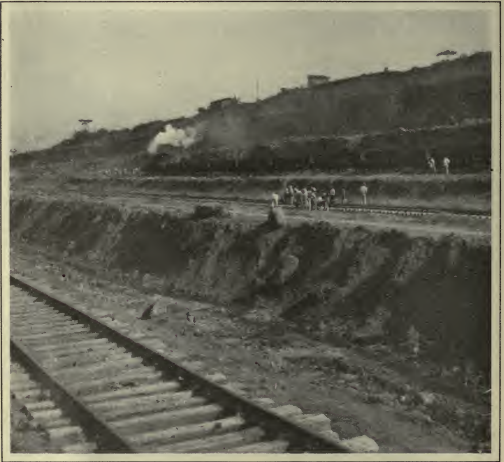
THE NORTHERN END OF THE CULEBRA CUT, Showing the lowest level reached in this section. There is still a distance of about ninety feet to go.
