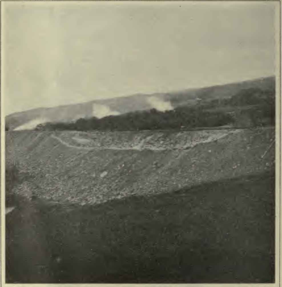
THE SINKING OF AN EMBANKMENT AT GATUN.
