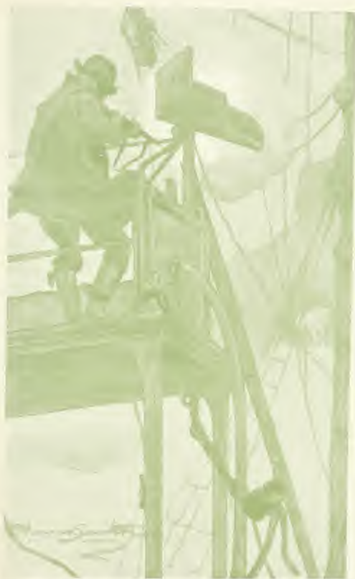
WORKING ON THE SCAFFOLDING OF THE PIPE, 1914.
