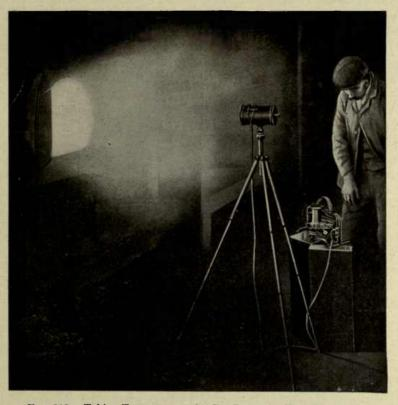
FIG. 219.-Taking Temperature of a Gas Retort by Féry Pyrometer.
