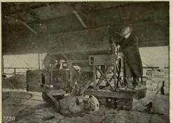
FIG. 58.-Coal Car ready for charging Producer.
