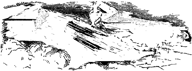
ICE-BELT BROKEN BY FALLING ROCK.
