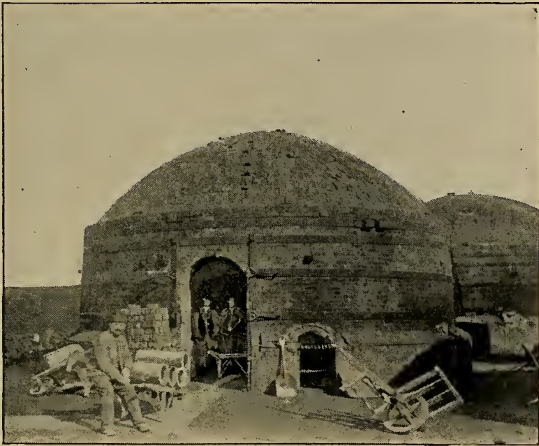
Circular down draft kiln for burning sewer pipe and drain tiles. J. Lyth & Sons, Angola.
