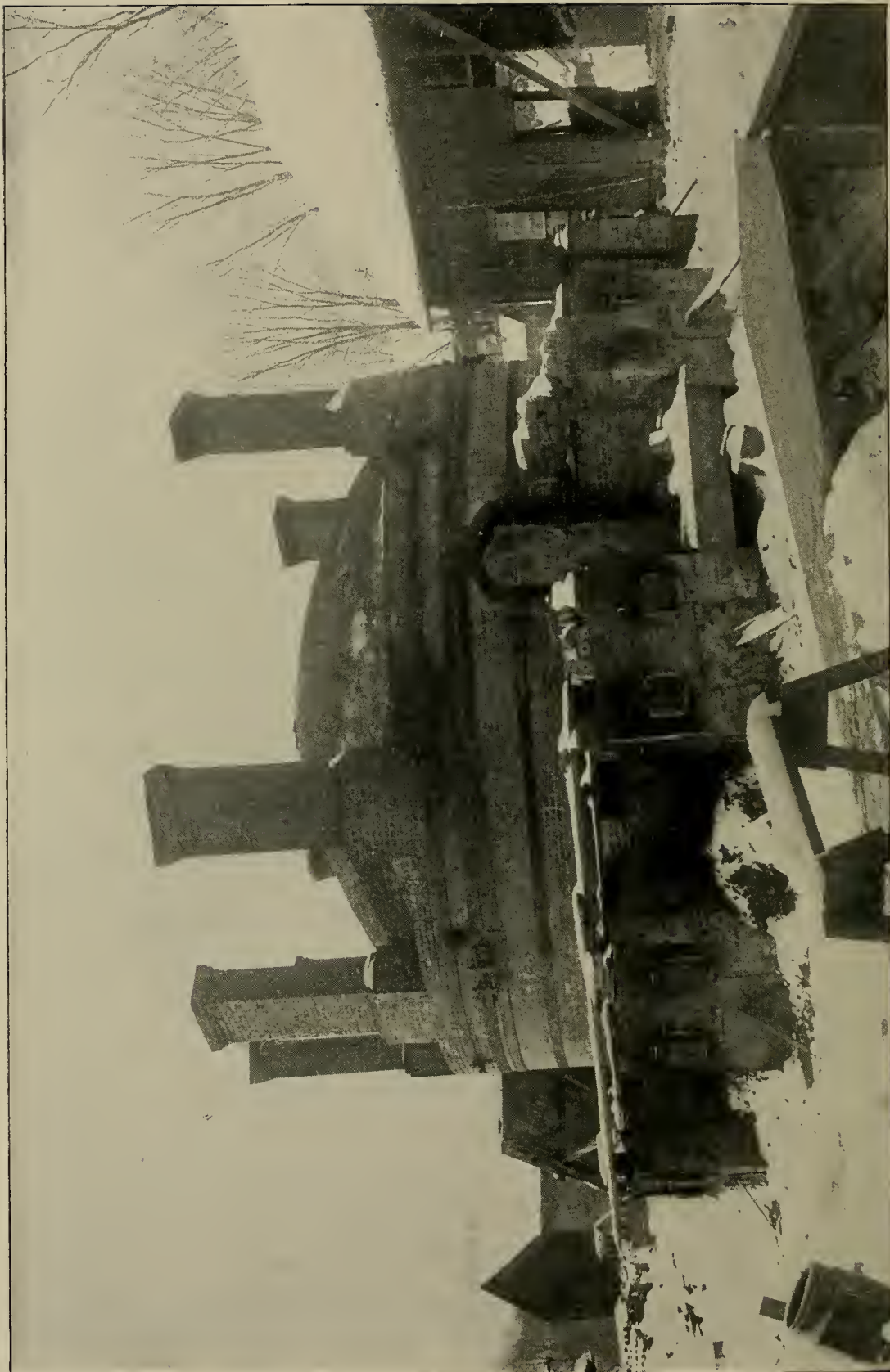
H. Ries photo. Grath coking furnace used for burning roofing tile. Celadon terra cotta co., Alfred Center.
