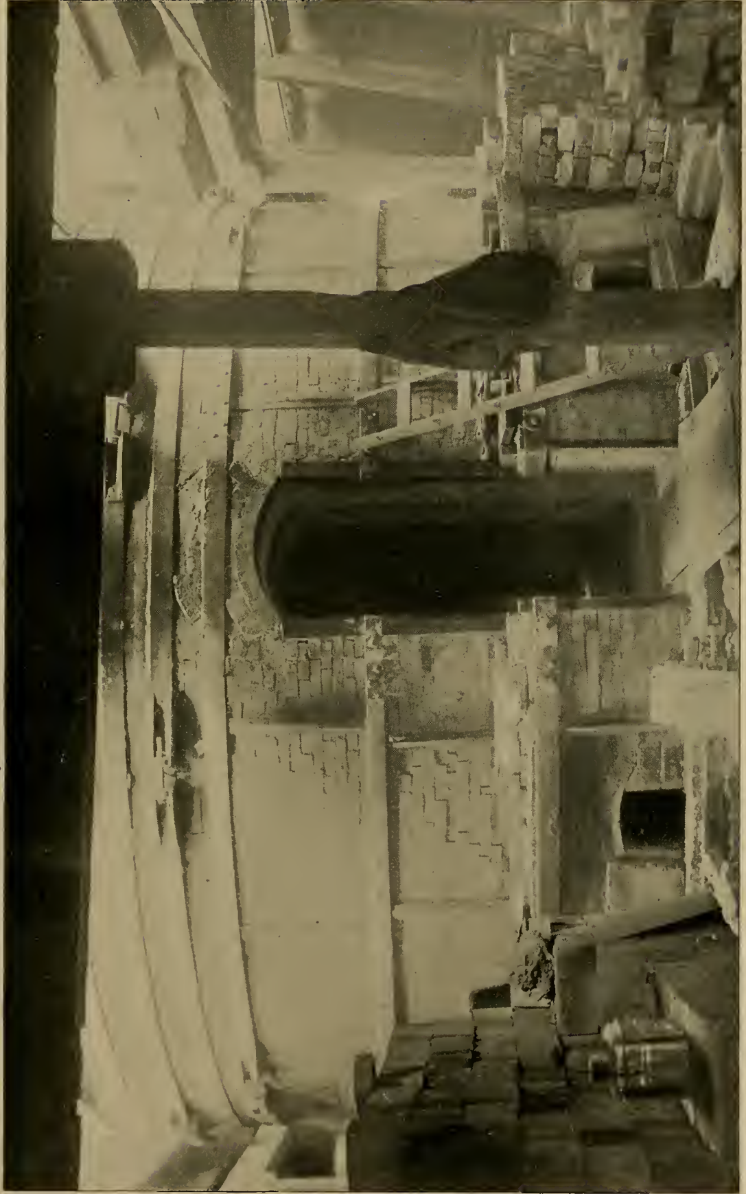
H. Ries photo. Circular down draft kiln used for burning fire brick. B. Kreischer's Sons, Kreischerville.
