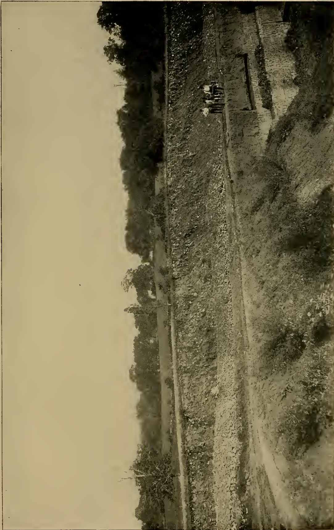
H. Ries photo. Unstratified material overlying clay at Meade & Co.'s bank, north of Low point.
