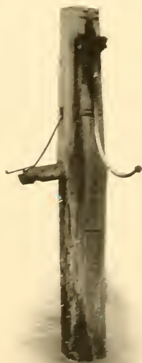
Old Street Pump
