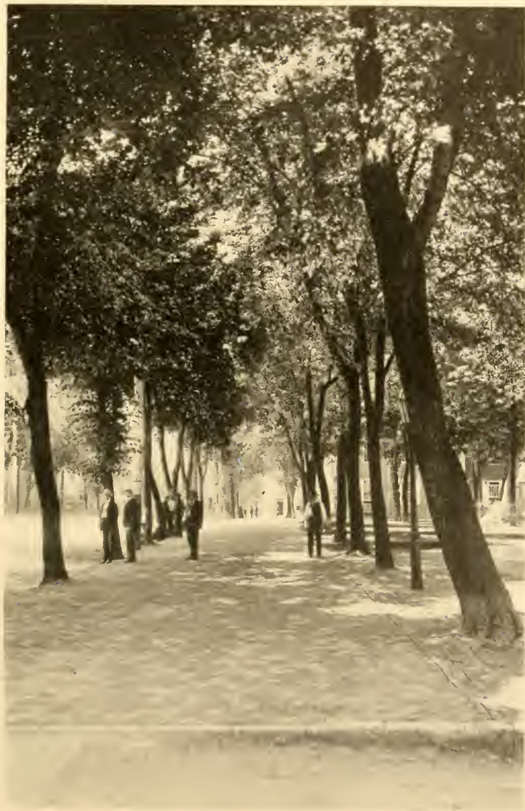
Hanover Street, Looking Southward
