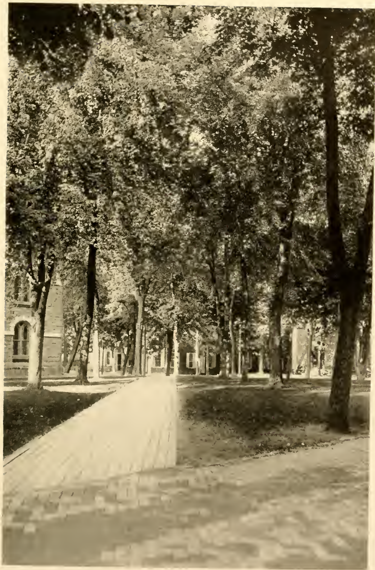
Public Square and Corner of First Presbyterian Church
