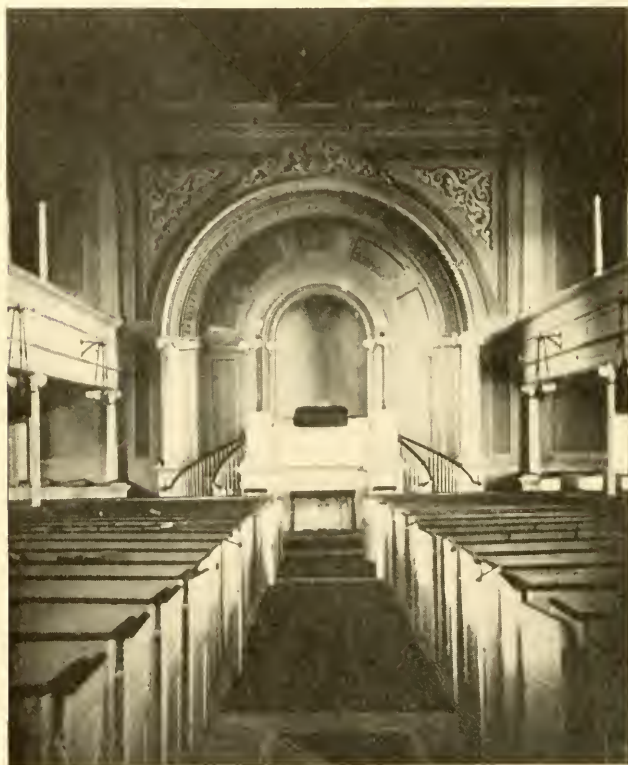
Interior of First Presbyterian Church. From 1827 to 1876
