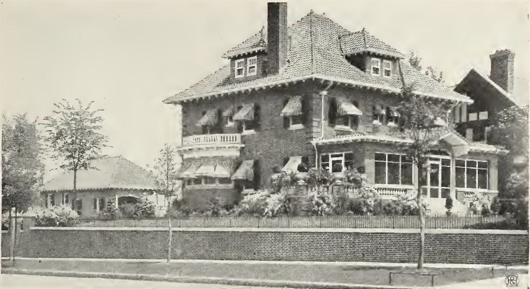
The retaining wall, topped with an artistic railing, and the pleasing shrub planting, give a distinct appearance of privacy.
