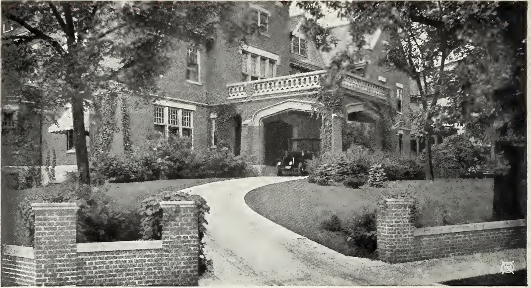
A skilful arrangement of shrubs with mature trees. Residence of F. E. Weyerhaeuser
