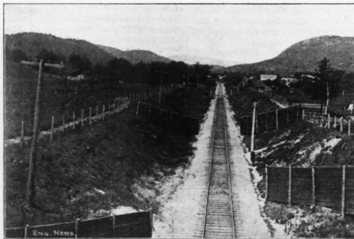
FIG. 4.—SNOW FENCES IN CUTS; BOSTON & MAINE R. R.
