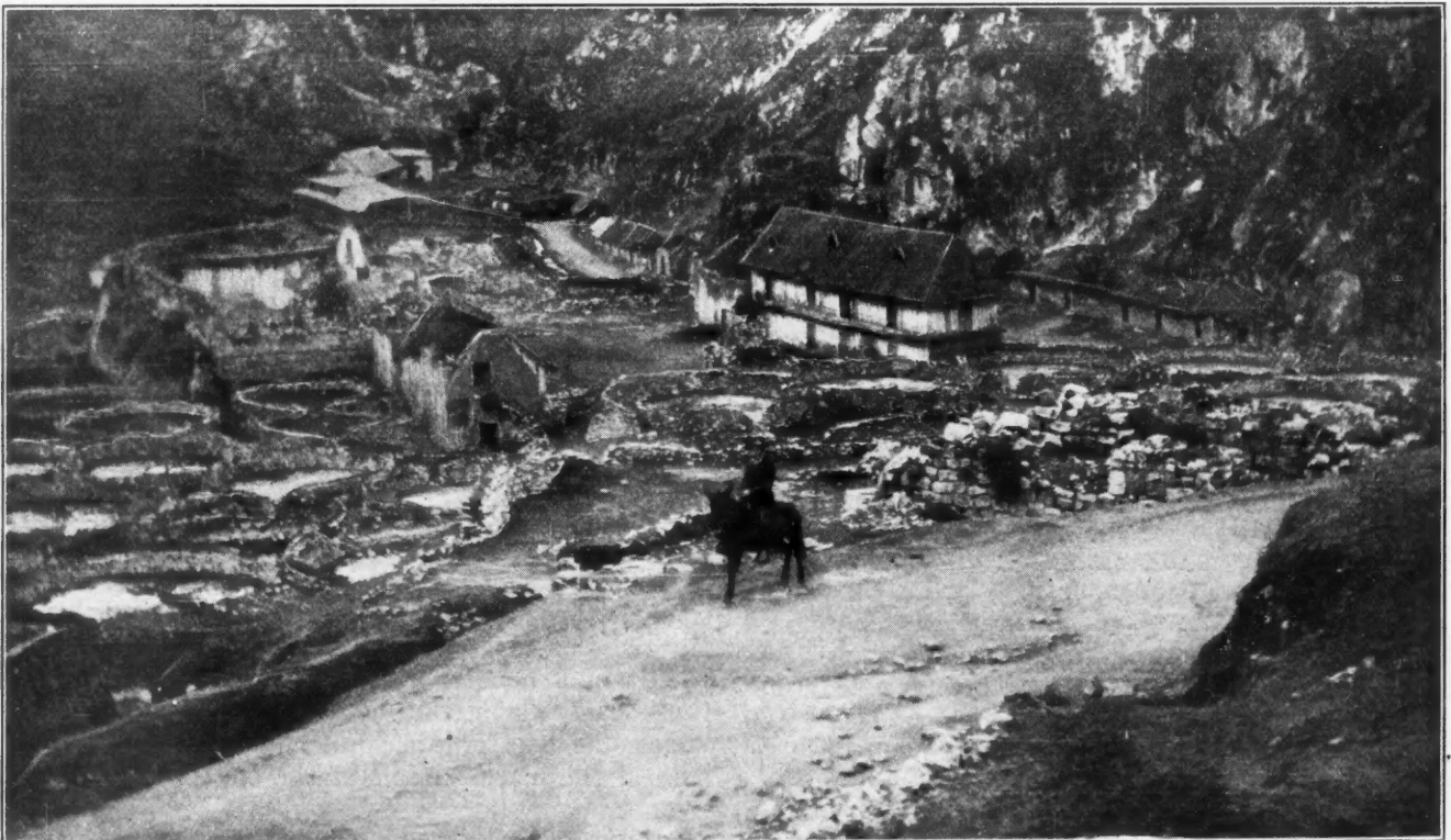
ABANDONED AMALGAMATION "PATIOS" NEAR CERRO DE PASCO, PERU
