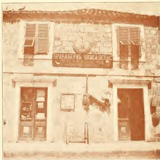
THE STRIPS OF STREETS A TYPICAL SHOP ON THE STRADONE, RAGUSA
