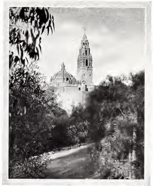
TOWER, CALIFORNIA BUILDING H. A. TAYLOR
