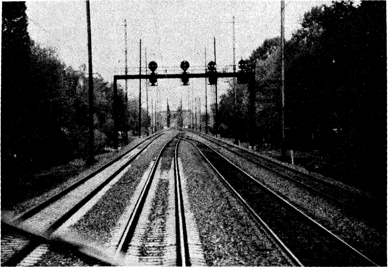
Figure 6. The northbound home signals at Gunpow as viewed from a northbound train moving at 125 mph on track 2. The aspect displayed for the train by signal 2N is "clear;" those displayed for the other tracks are "stop." From left to right, the tracks are 3, 2, 1, and A.
