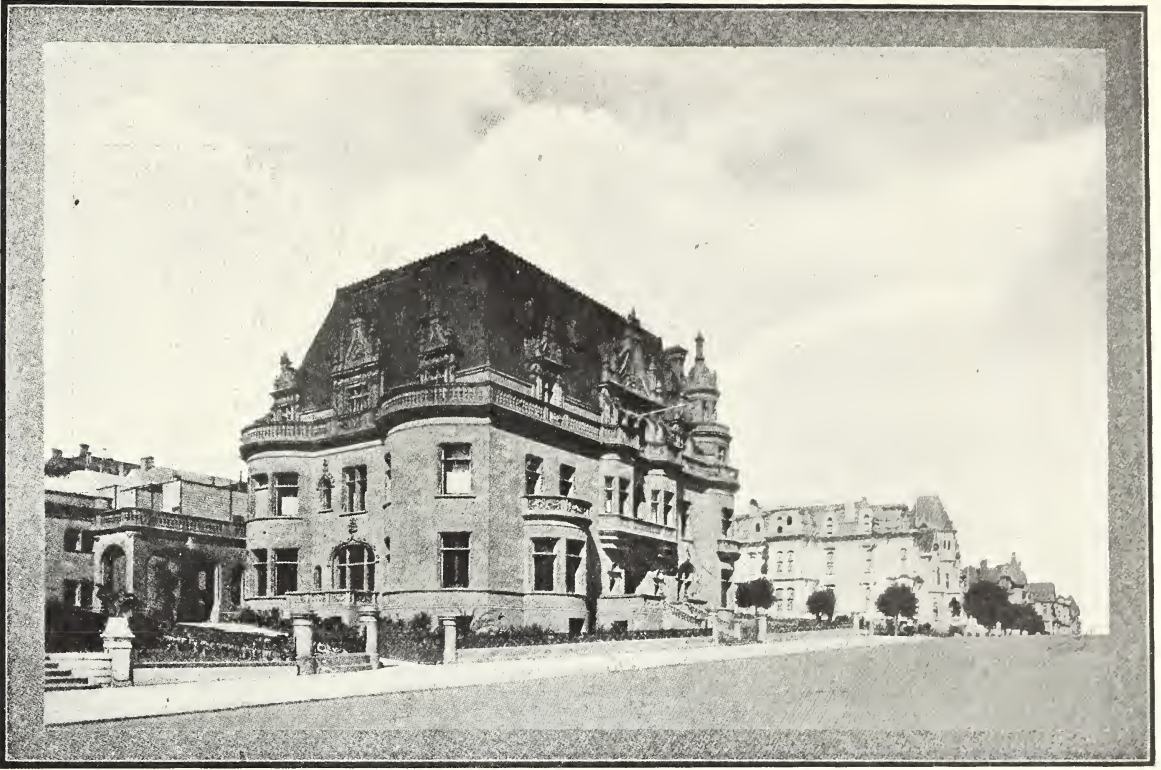
A VAN NESS AVENUE RESIDENCE, SAN FRANCISCO, BEFORE THE DISASTER.
