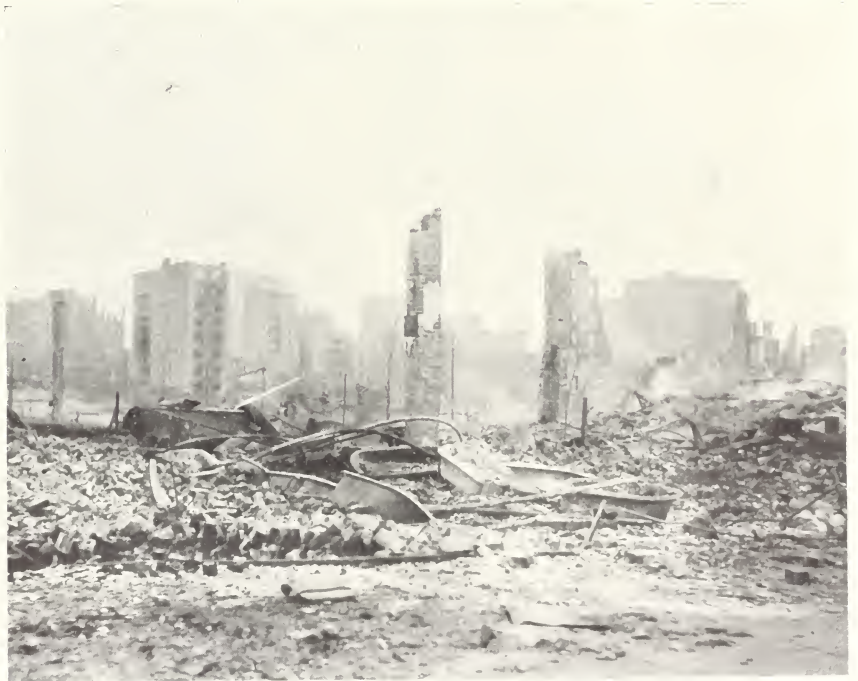
VIEW OF THE SITE OF THE BALDWIN ANNEX, TAKEN ON MARKET STREET, LOOKING NORTHEAST
