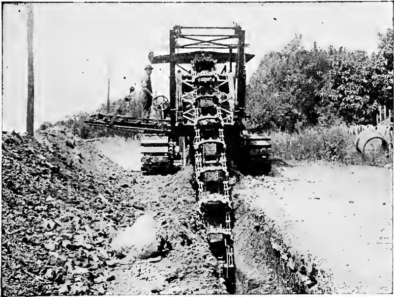
FIG. 61.—LADDER-DREDGE TYPE OF TRENCH EXCAVATOR.
