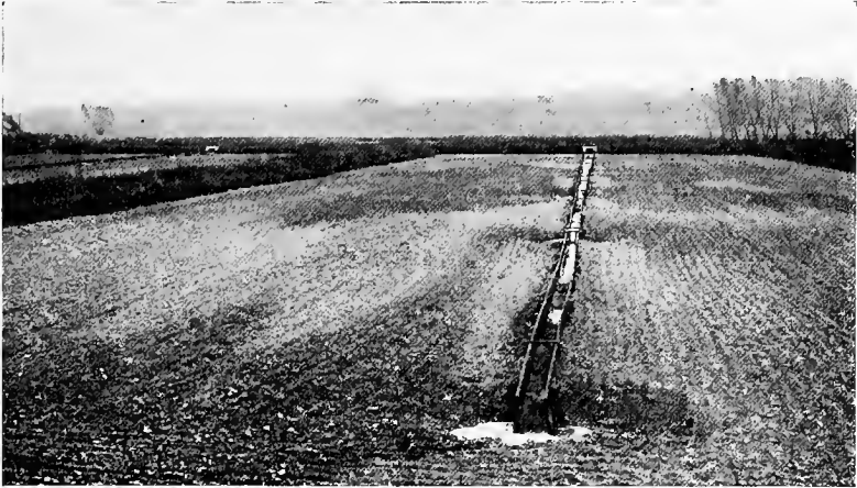
FIG. 69.—ARTIFICIAL SAND FILTER WITH WOODEN DISTRIBUTOR.
