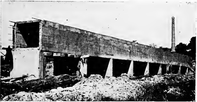
FIG. 14.—OUTFALL SEWER CROSSING VALLEY ON HYDRAULIC GRADIENT.
