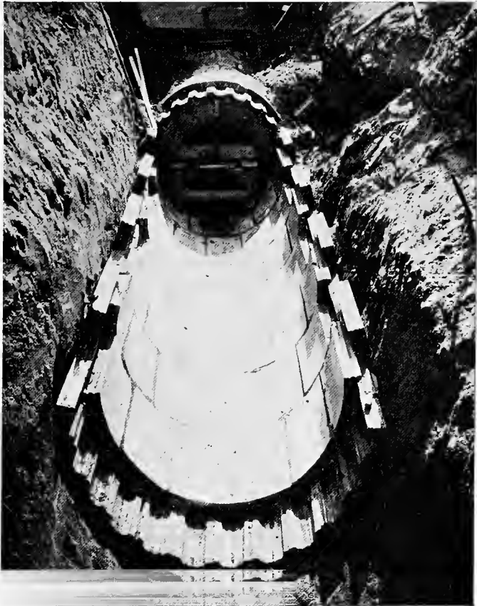
—FIFTY-EIGHT-INCH CIRCULAR BRICK SEWER AT WAUSAU, WIS.
