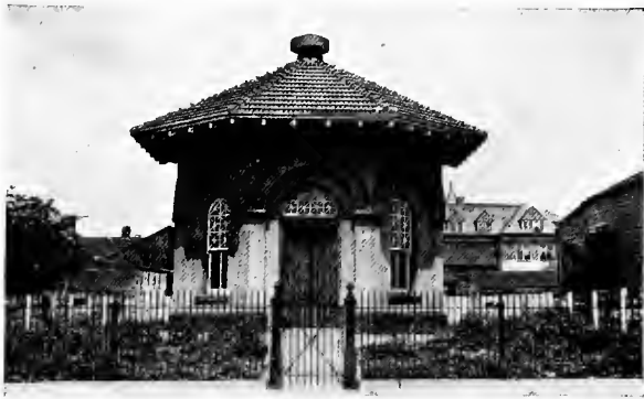
FIG. 16.—NEW ORLEANS PUMPING STATION SUPERSTRUCTURE.
