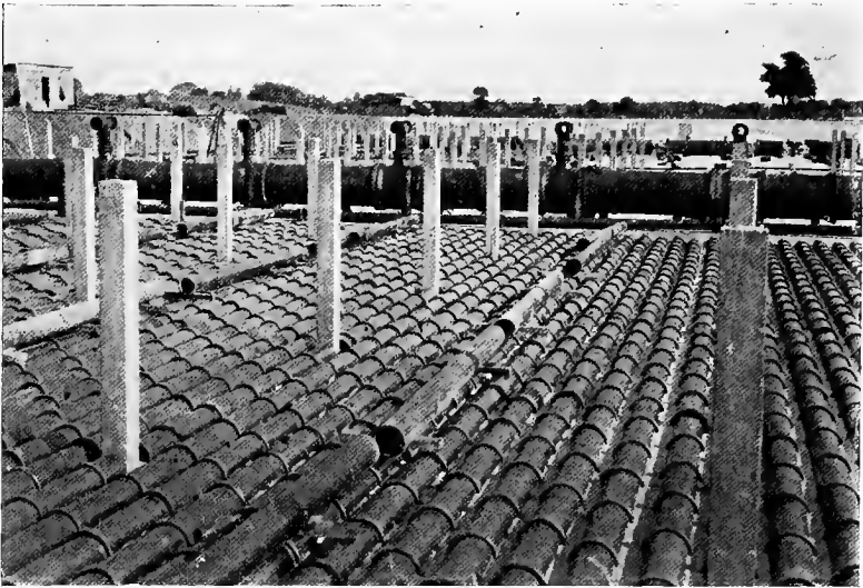
FIG. 74.—SPRINKLING FILTER DRAINAGE SYSTEM.
