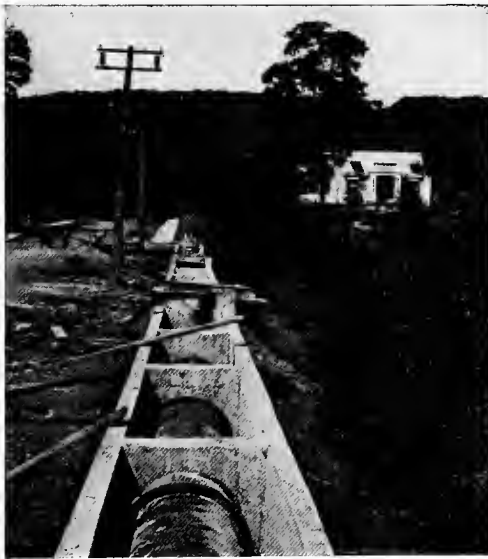
FIG. 1. INVERTED SIPHON ON GRADIENT ABOVE STREET SURFACE. THE PIPE IS ABOVE WALL ALONG THE SIDE OF A FILL ACROSS VALLEY.
