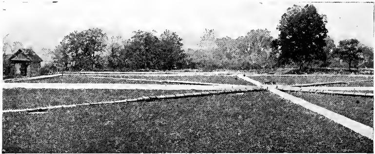
FIG. 72.—CONTACT BEDS WITH TILE PIPE DISTRIBUTORS AND HAND GATES.
