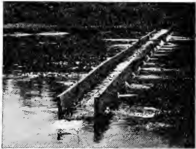
FIG. 70.—WOODEN TROUGH DISTRIBUTOR IN ACTION.
