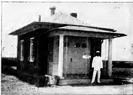
FIG. 80.—NEAT SEWAGE TREATMENT HOUSE Screening and disinfecting plant at Atlantic City.
