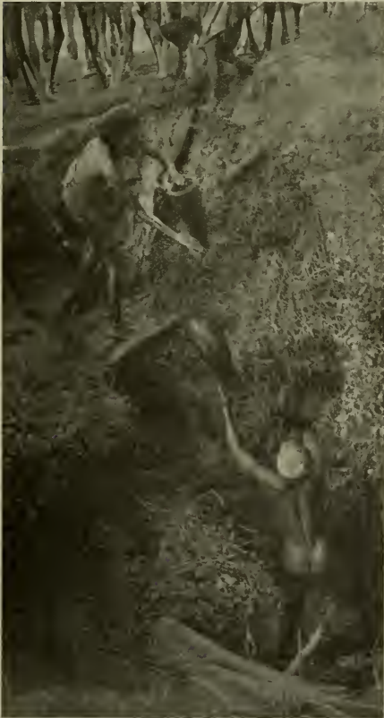
Some of the Somali wells are eighty feet deep and require at least eight natives supported one above the other on steps along the walls of the well, to pass the water in wooden buckets ( chatties ) to those waiting at the top
