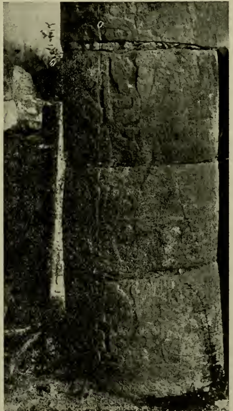
Sculptured column made of drum-shaped sections — South Temple of the Ball Court. The designs represent warriors, reclining figures and a wealth of highly conventionalized serpent heads
