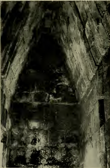
Typical vaulted room illustrating the architectural skill of the Maya builders. The vault is a solid concrete mass covered by a veneer of nicely cut facing stones
