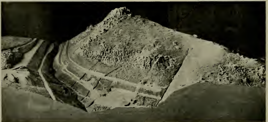
One section of Copper Queen Mine model, showing the surface of clay modeled upon the wooden core. It is ready for making the mold from which to cast the final surface in plaster
