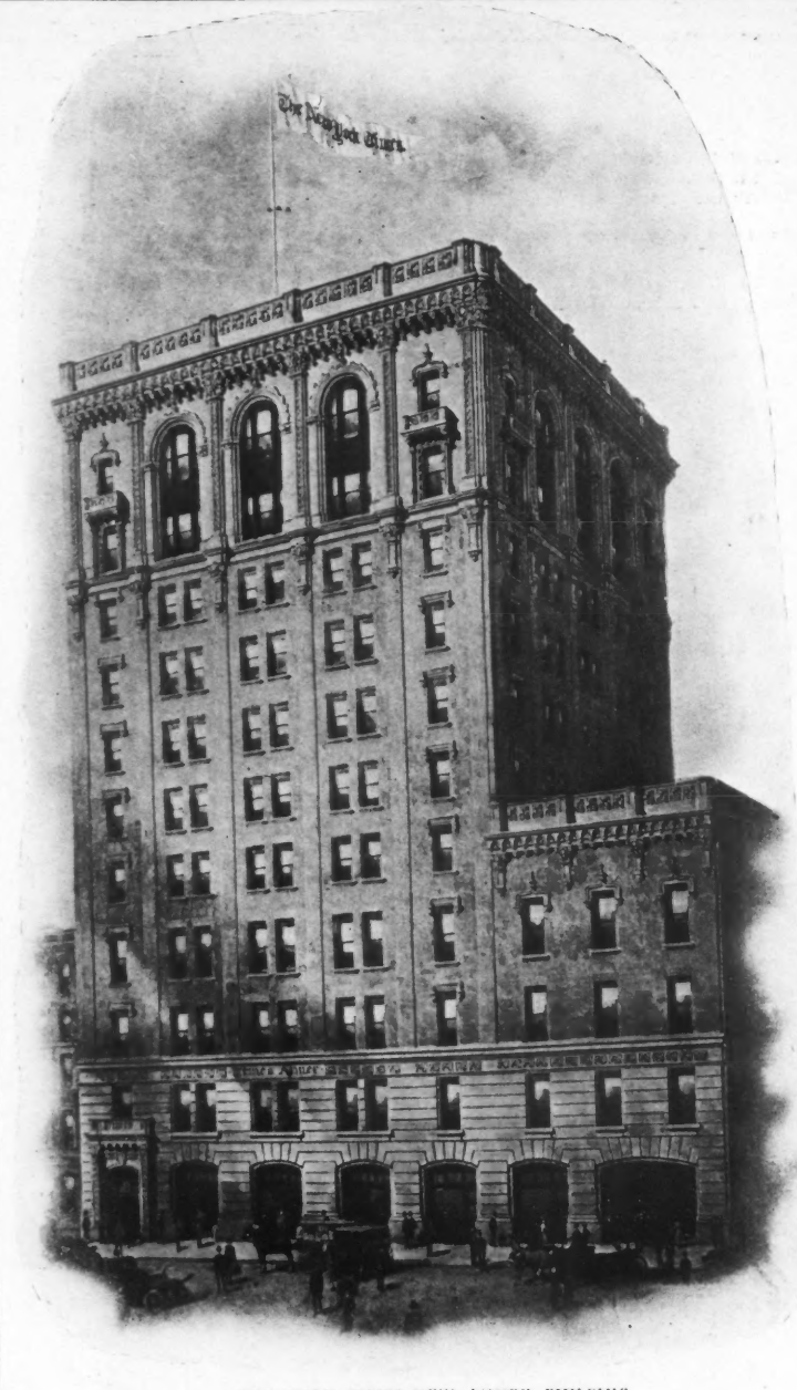
NEW YORK TIMES NEW ANNEX BUILDING.
