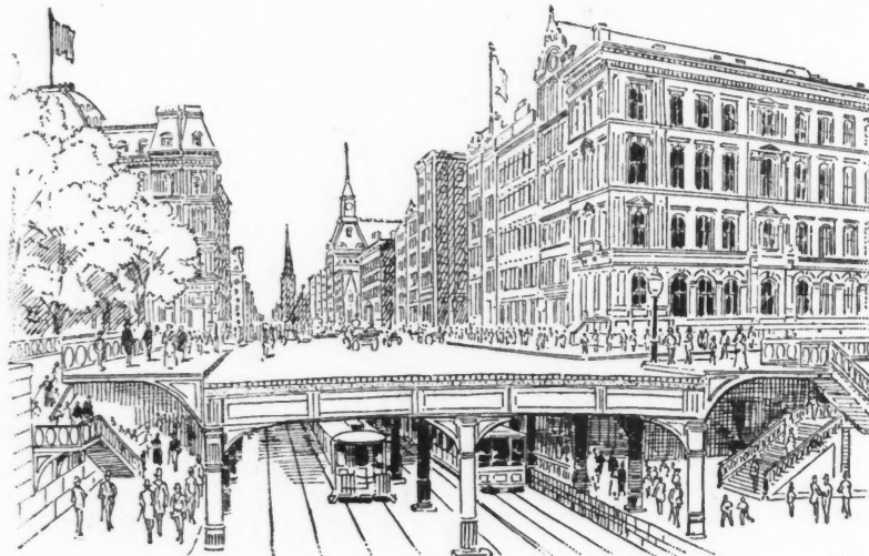
RAPID TRANSIT FOR NEW YORK; THE FOUR-TRACK TUNNEL.
