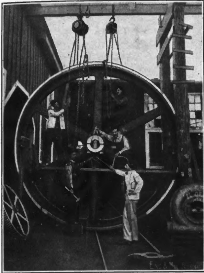
FIG. 2. HEAVY DRIVE WHEEL REBORED AT MINE
