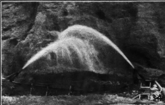
1 and 2. A 4-in. giant with water at 125-lb. pressure attacking frozen gravel forming the mountain side 3. View showing height of gravel bank and trestle carrying pipe line 4. Hydraulicking the frozen gravel with water brought from another watershed through a pipe line 60 miles long 5. Main sluice box, showing riffles of 12-in. cubes of wood, set on end 6 and 7. The creek bottom was first dredged and the wagon road established on dredge tailings; to the right is a nearer view of the extensive cribbing used in protecting the wagon road from the hydraulic tailings; the telephone poles have been reset three times
