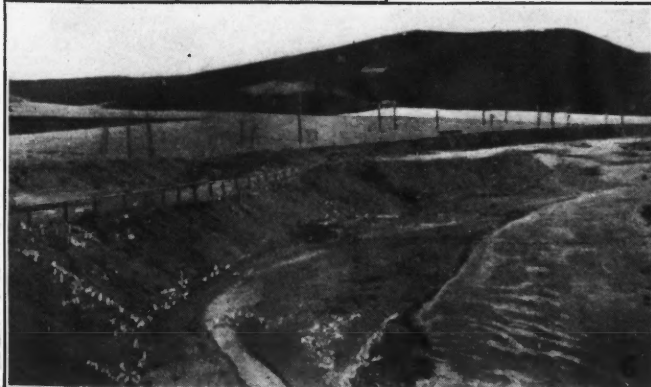
1 and 2. A 4-in. giant with water at 125-lb. pressure attacking frozen gravel forming the mountain side 3. View showing height of gravel bank and trestle carrying pipe line 4. Hydraulicking the frozen gravel with water brought from another watershed through a pipe line 60 miles long 5. Main sluice box, showing riffles of 12-in. cubes of wood, set on end 6 and 7. The creek bottom was first dredged and the wagon road established on dredge tailings; to the right is a nearer view of the extensive cribbing used in protecting the wagon road from the hydraulic tailings; the telephone poles have been reset three times
