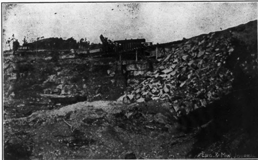
STEAM SHOVEL REMOVING OVERBURDEN AT A SOUTH DAKOTA GOLD MINE
