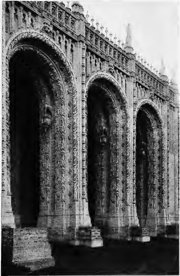
DETAIL FROM THE COURT OF ABUNDANCE LOUIS CHRISTIAN MULLGAEDT, ARCHITECT
