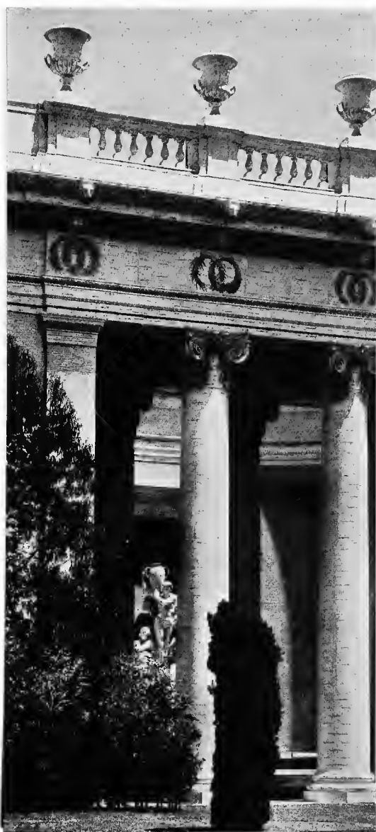
NICHE DETAIL FROM THE COURT OF THE FOUR SEASONS HENRY BACON, ARCHITECT
