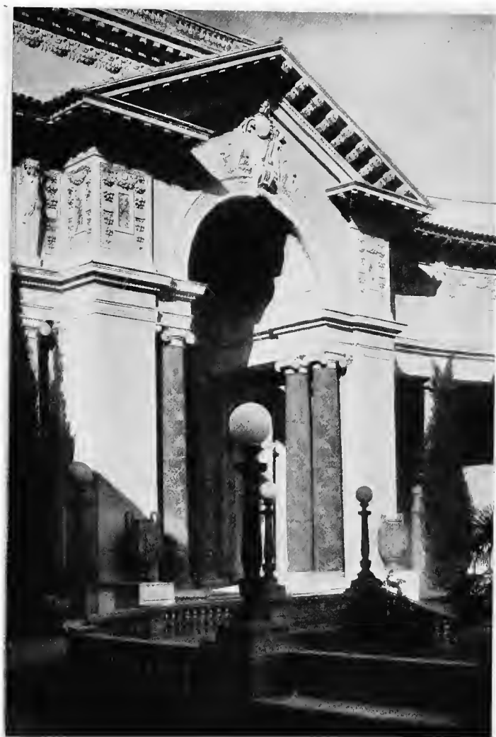
NORTHERN DOORWAY IN THE COURT OF PALMS GEORGE W. KELHAM, ARCHITECT
