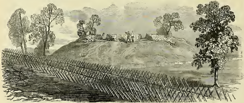
RUINS OF A CONFEDERATE FORT ON THE SOUTHEAST OF ATLANTA, WITH CHEVAUX-DE-FRISE AND ABATIS IN FRONT.
