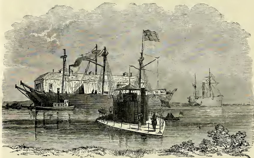
ADMIRAL DUPONT'S MACHINE-SHOP IN CHARLESTON HARBOR, S. C.
