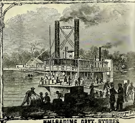
UNLOADING GOVT. STORES
