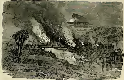
BURNING CONFEDERATE STOREHOUSES.
