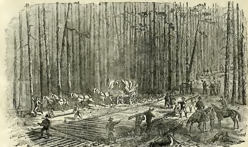
BUILDING A CORDUROY ROAD IN THE WOODS, NEAR THE WELDON RAILROAD, VA.
