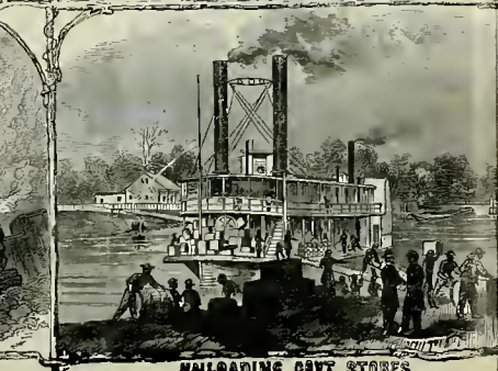
UNLOADING GOVT. STORES
