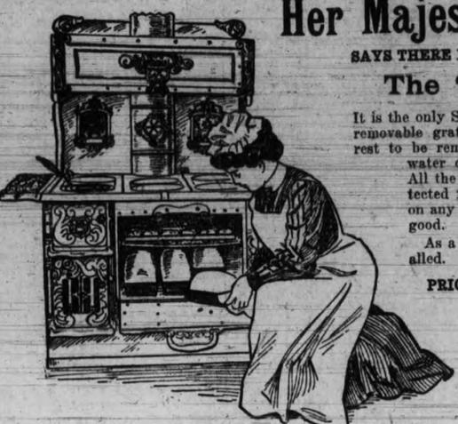
It is the only Steel Range made with a patent removable grate support, allowing the brick rest to be removed without running off the water or disturbing the water-front. All the exposed parts of steel are protected from the fire. There is no top on any Range just as strong, plain and good. As a Cooking Apparatus it is unrivalled.
