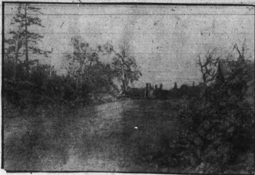
ROCK CUT ON LINDEN AVENUE.
