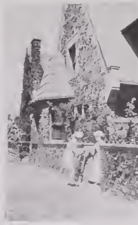
Parting at the Gate S 2133
