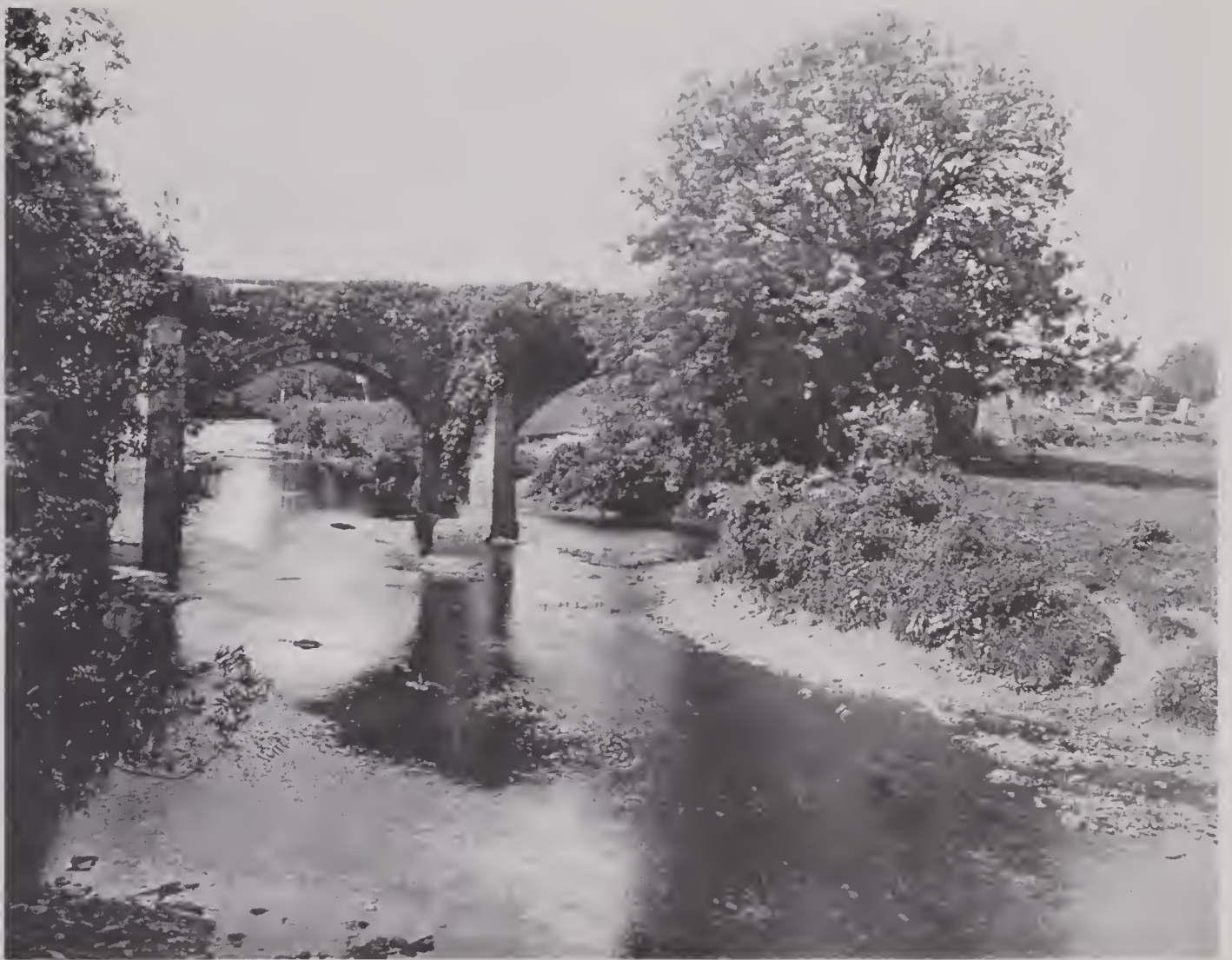
Under Ivy Bridge
