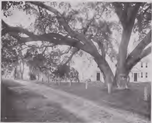
The Protecting Home Tree C and E 1517
