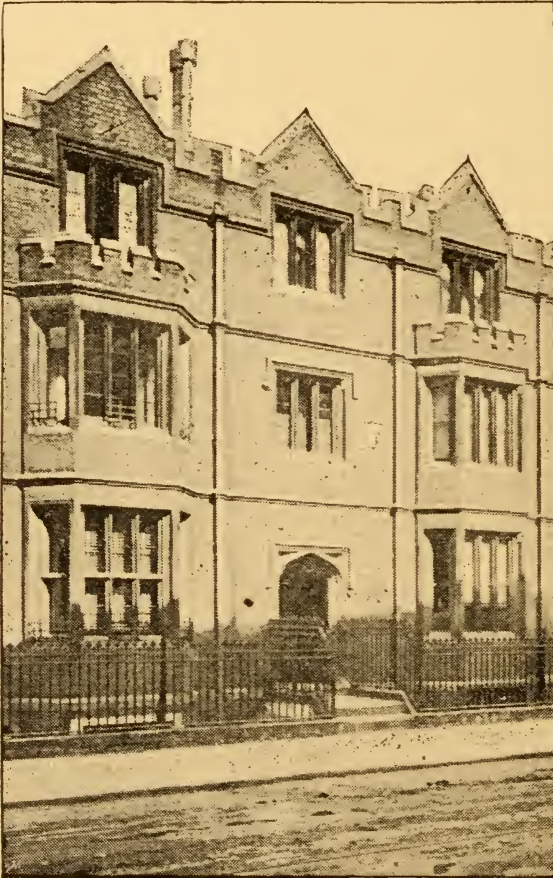
TENNYSON'S ROOMS, CORPUS BUILDINGS.
