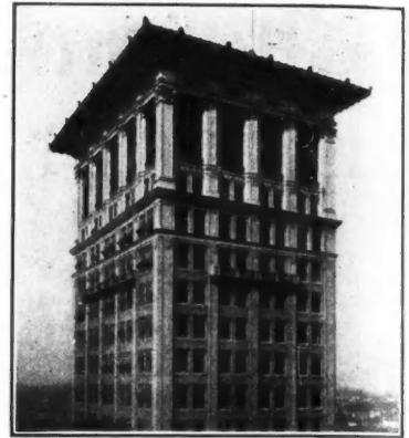
Combination of copper cornice, terra-cotta crowning detail with iron infilling standing upon a brick shaft. This combination of materials working out in perfect harmony and creating a building of most distinctive character. Richmond, Va. Alfred C. Bossom, Architect.
