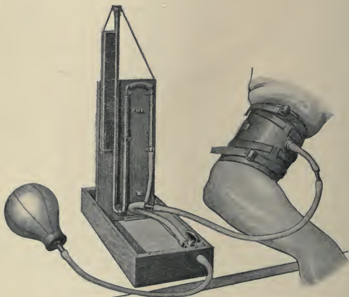
FIG. 5.—Janeway's sphygmomanometer, attached to arm, showing method of retention of cuff, arrangement of manometer, with Politzer bag inflator.
