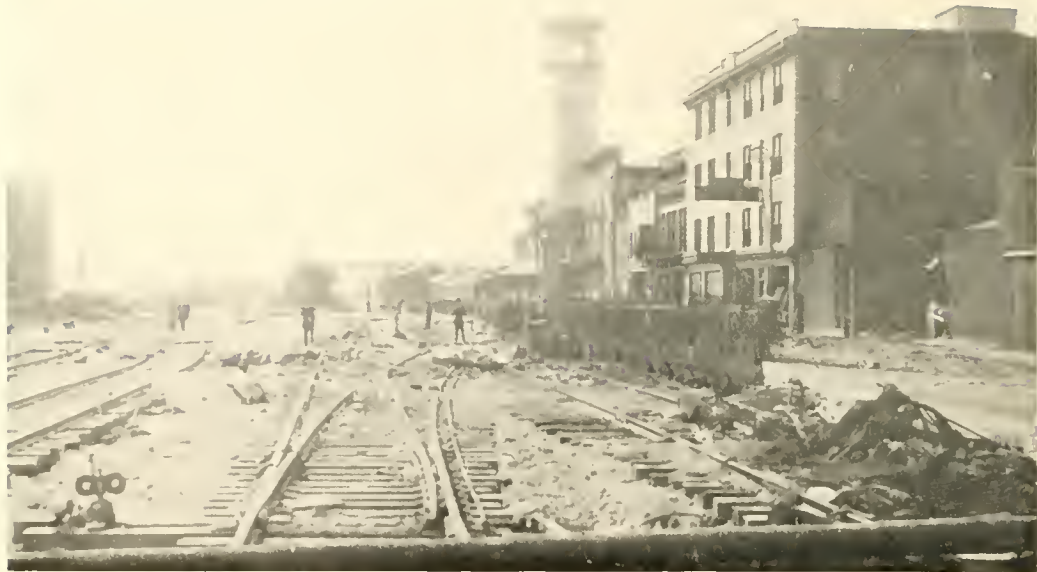
WASHOUT of TRACKS at UNION DEPOT
