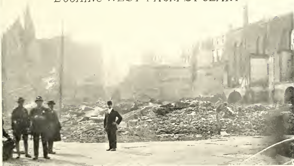
VIEW OF FIRE ZONE LOOKING WEST FROM ST CLAIR
