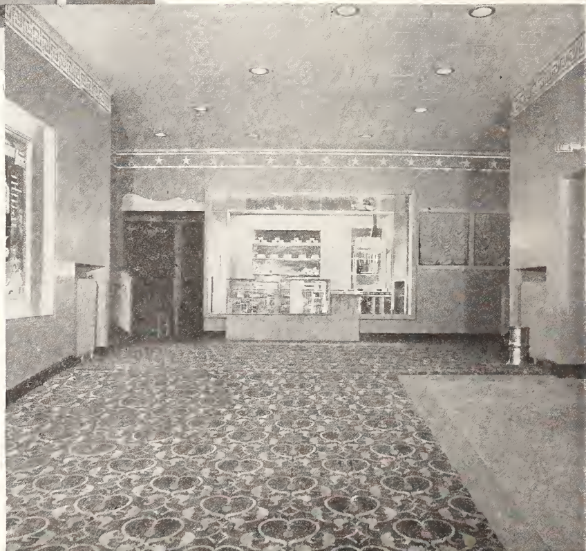
Carrara architectura glass framing aluminum display cases and window of inside box-office obliterated the original entrance area. Below is the lobby toward auditorium before alterations, at right as remodeled.
