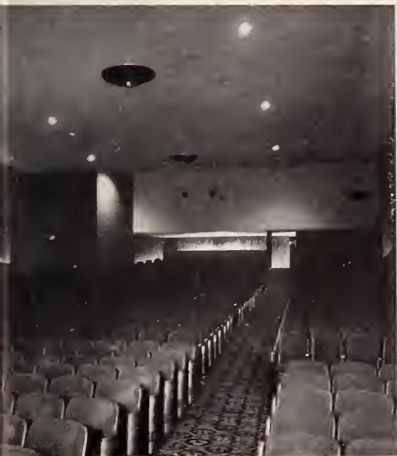
The auditorium — toward the stage (right) and toward the standee space (above), compared with the original plan and treatment in similar views. The side wall panels are covered in deep blue velour and are lighted by blue neon concealed in the top of the dado. The ceiling is acoustical plaster painted off-white. Seating is now on one floor.
