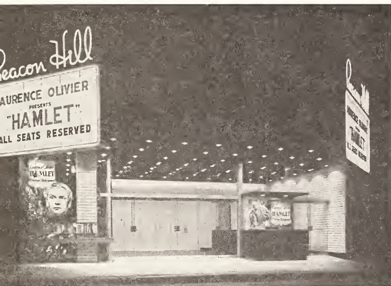
New front and vestibule of the Beacon Hill.
