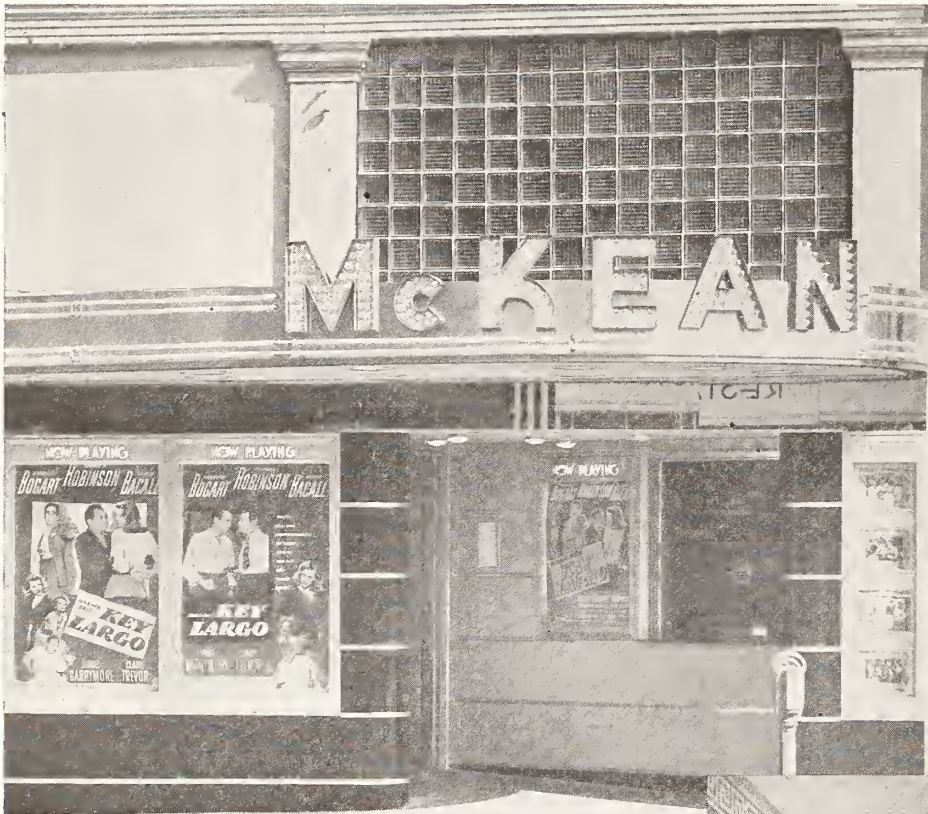
Carrara architectura glass framing aluminum display cases and window of inside box-office obliterated the original entrance area. Below is the lobby toward auditorium before alterations, at right as remodeled.
