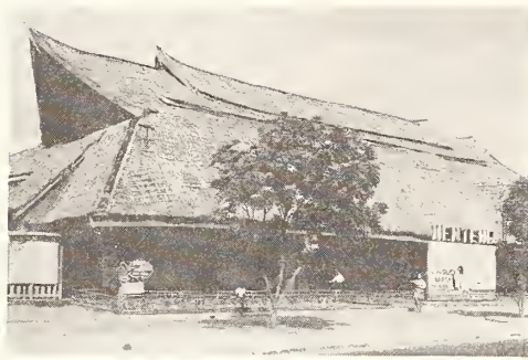
Theatre design in Java. This 1,000-seat motion picture house in Batavia is constructed of bamboo, except for a brick projection room. Measuring 114x54 feet, it was built in six weeks. Walls are of bamboo matting, the roof of sago-palm leaves.
