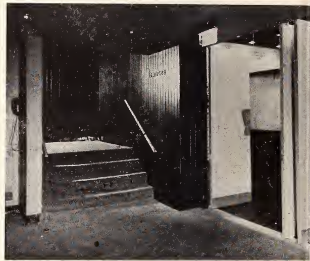
Sections of the foyer as modernized, compared with the original in before-remodeling views of the same areas. The lounge corner is faced in mahogany-stained vertical boarding. Birch plywood is also used for the walls.
