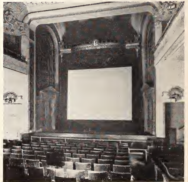
The old-fashioned auditorium, with balcony extensions along the sides to aggravate the problem presented by its heavy ornamental treatment, was modified principally by a process of obscuration rather than structural changes. What ornament could not be readily removed, was "cleaned up" with paint, dark blue and light gray being used for walls, dark blue for the ceiling.
