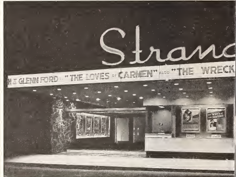
New front and entrance of the Strand in Thompsonville.
