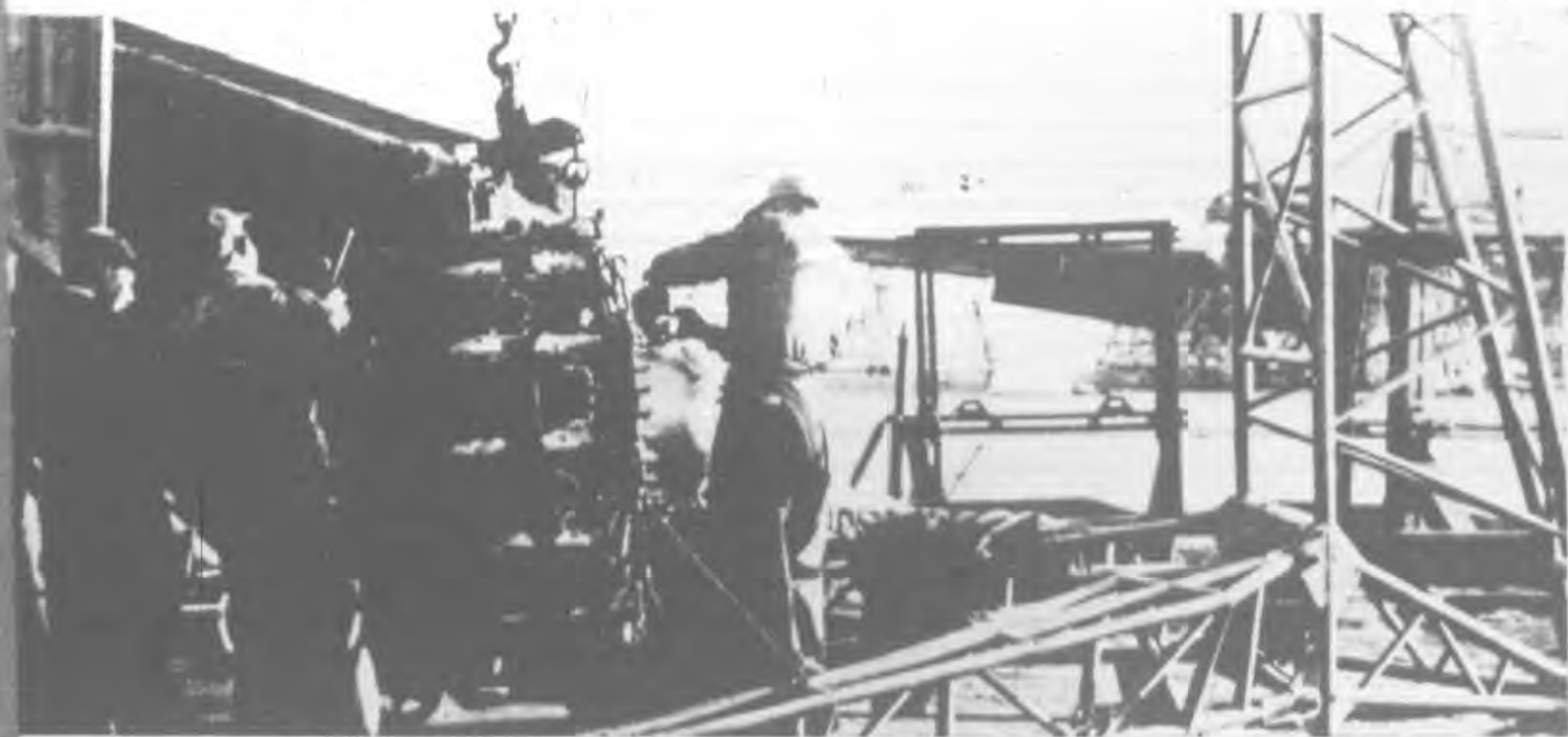
POWER PLANT —Powerful engine from salvage C-54 is dismantled while hanging from crane at CAT's Tien Ho workyard.
