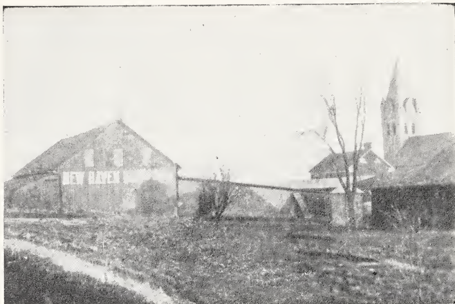
View of Our Storage Sheds
