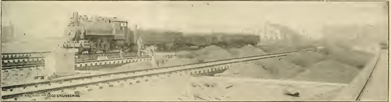
COAL STORAGE UNDER WATER. APPEARANCE OF THE BIN BEFORE BEING FLOODED.
