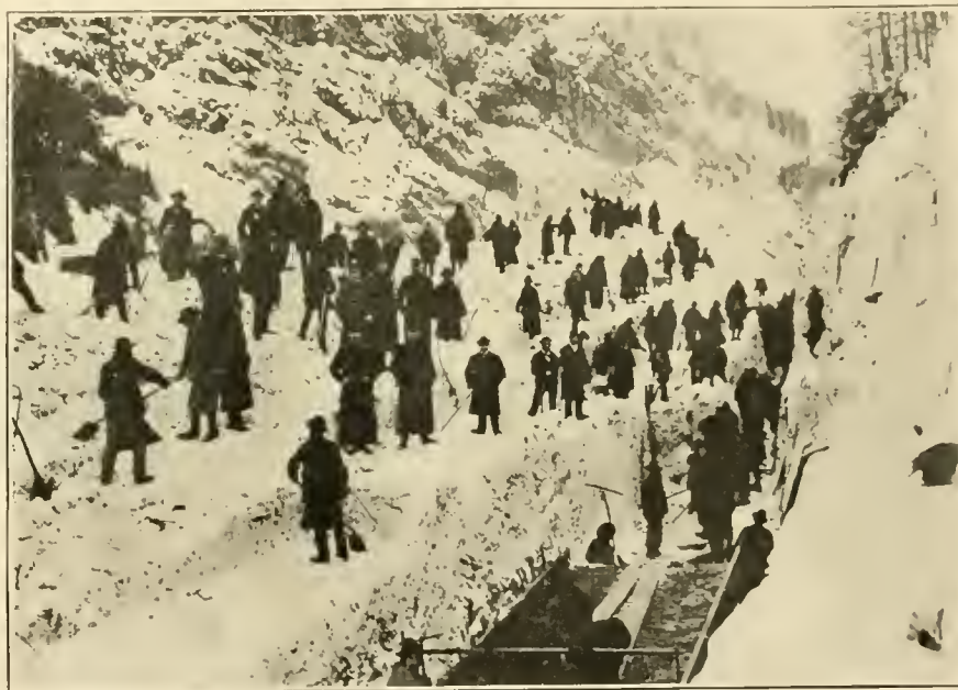
AVAILANCHE ON A RAILWAY LINE ON THE AUSTRO-ITALIAN FRONTIER.
