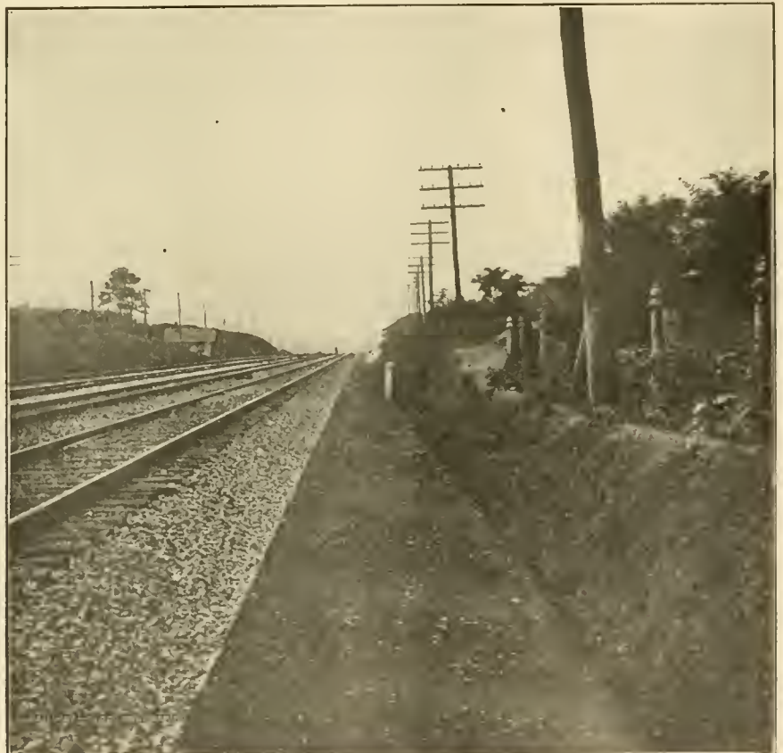
WELL KEPT AND CLEAN SIDE DITCH.
