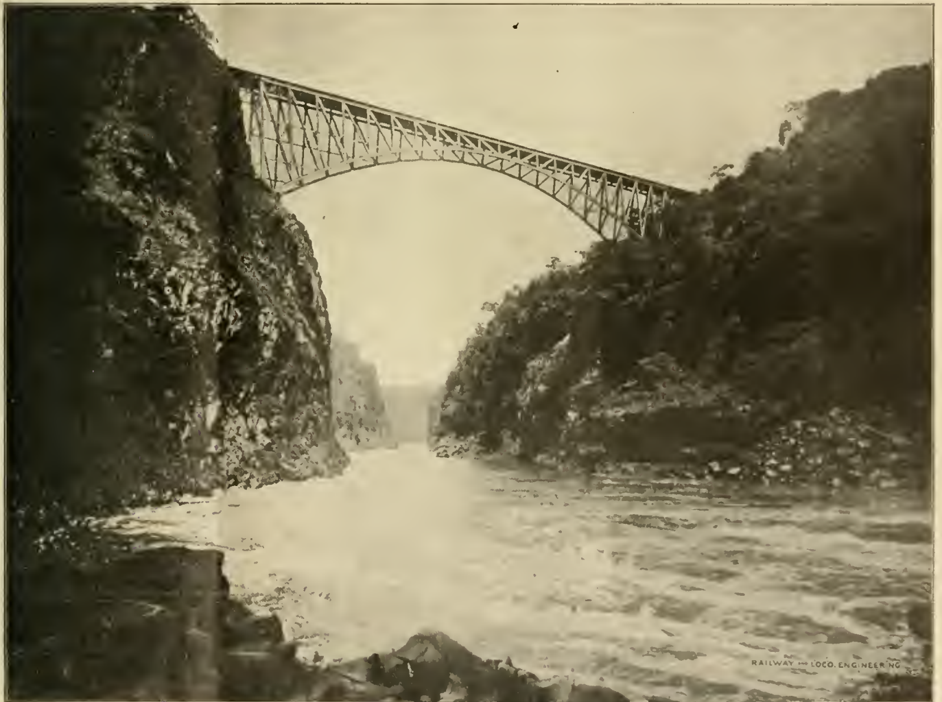
STEEL ARCH OVER THE ZAMBESI RIVER ON THE CAPE-TO-CAIRO RAILWAY.
