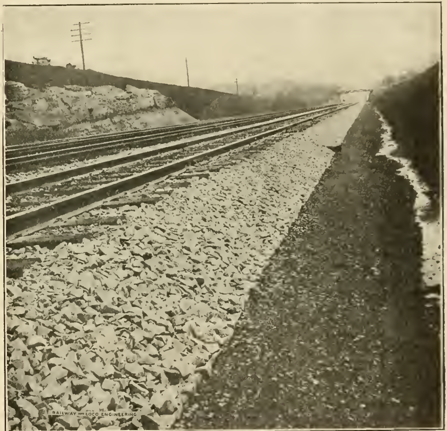
WELL DRAINED PENNSYLVANIA TRACK.
