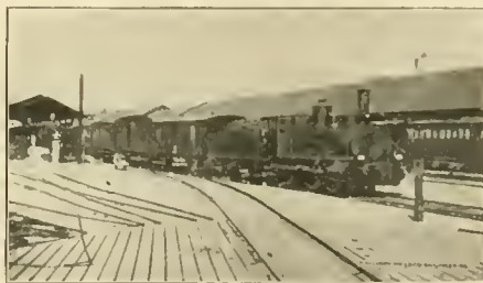
STATION AT BASLE, SWITZERLAND.
