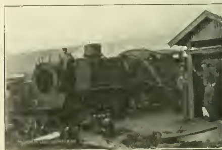
RAILS SPREAD ON A CURVE.
