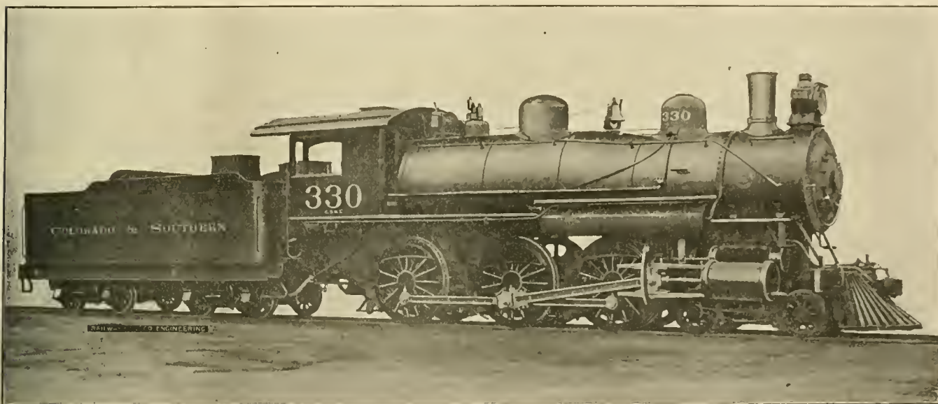
SIMPLE TEN-WHEEL ENGINE FOR THE COLORADO &amp; SOUTHERN.
