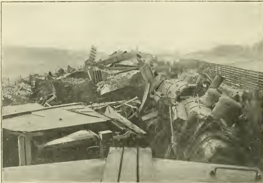
RESULT OF A SHORT BRAKE PIPE.
