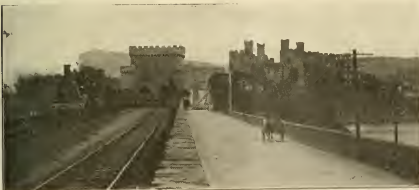
ENTRANCE TO RAILWAY TUBULAR BRIDGE AT CONWAY CASTLE.
