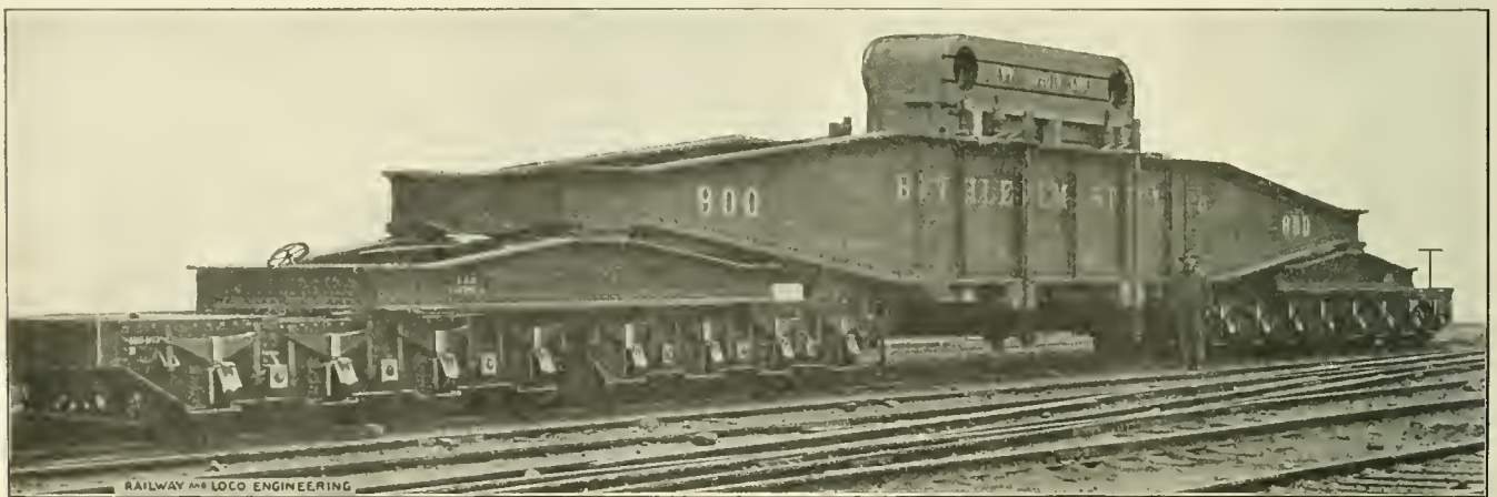
SPECIAL ONE HUNDRED-AND-FIFTY TON STEEL FREIGHT CAR.
