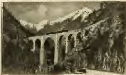
SAINT MARY'S VIADUCT, CHAMOUNIX.
