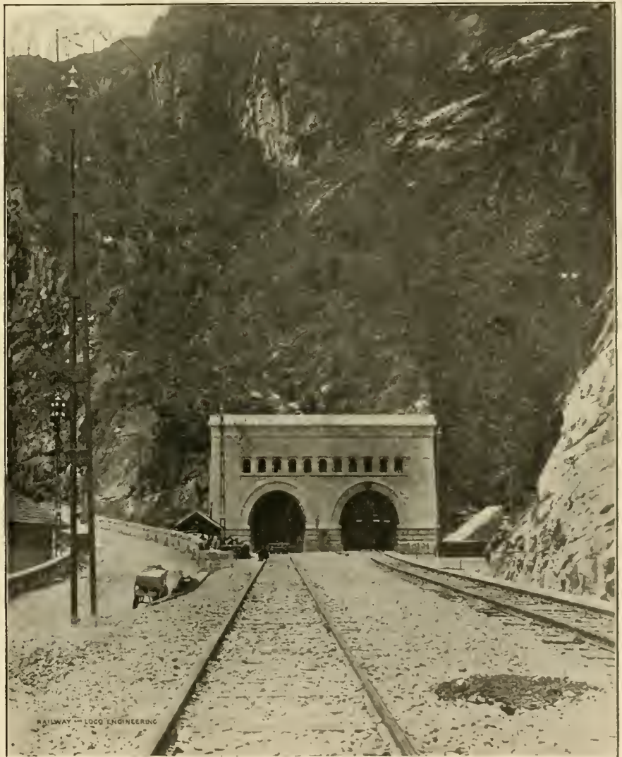
PORTAL ON THE ITALIAN SIDE AT DOMO D'OSSOLA. ENTRANCE TO BOTH TUNNELS CLOSE TOGETHER.
