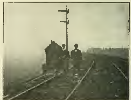
FIG. 1. TRIPPER ON THE TRACK.
