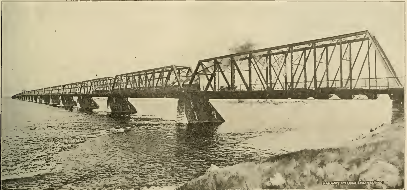
VICTORIA JUBILEE BRIDGE OVER THE ST. LAWRENCE ON THE PIERS OF THE OLD TUBULAR BRIDGE.
