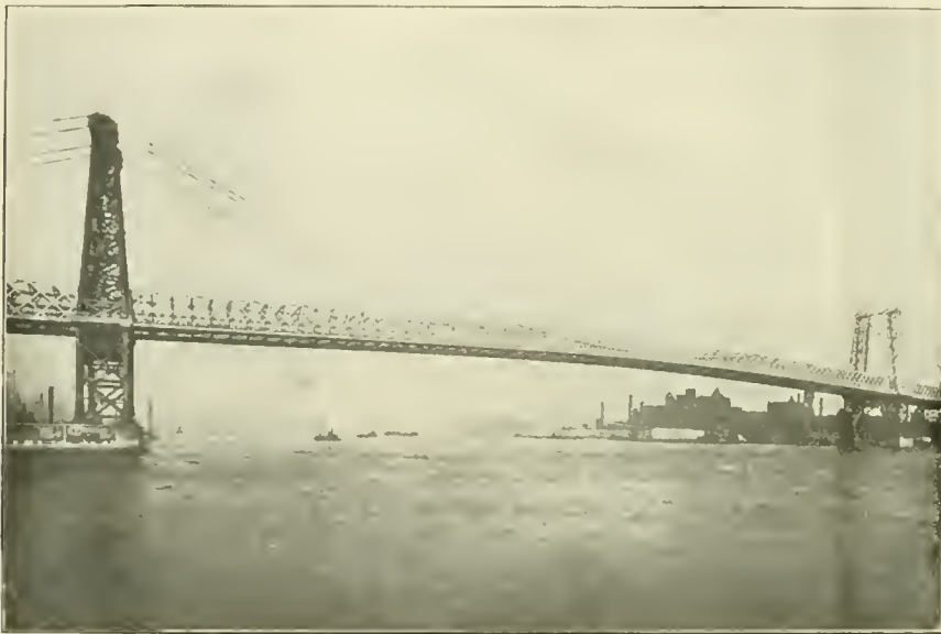
WILLIAMSBURG SUSPENSION BRIDGE, NEW YORK.
