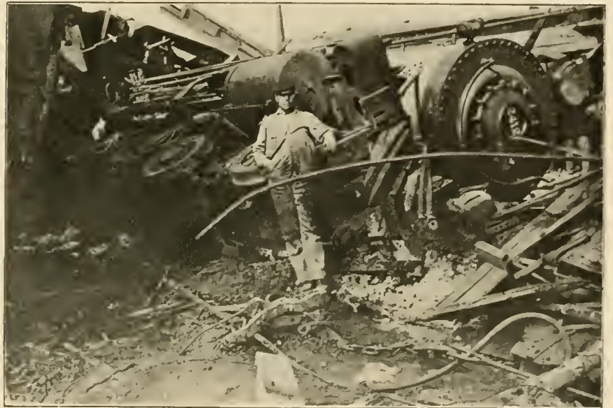
WAITING FOR THE WRECKING CREW.
