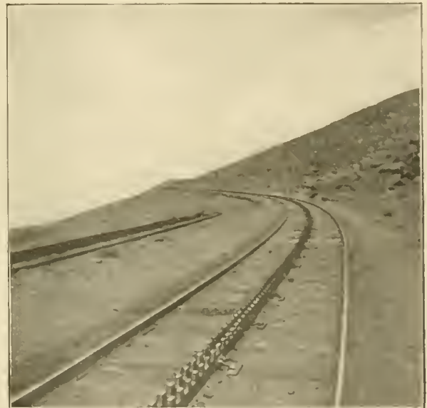
PIKE'S PEAK RAILWAY, SHOWING RACK RAIL.
