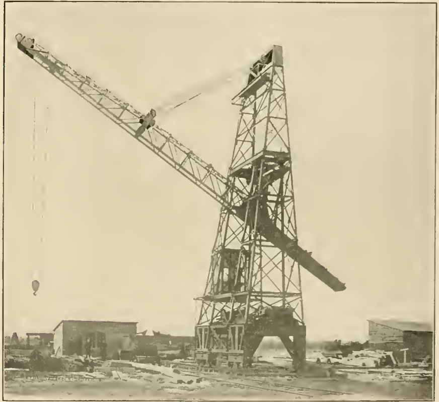
FIG. 1. WORKING POSITION OF TRAVELING CRANE.
