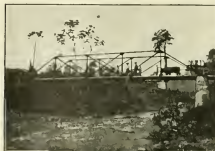
BRIDGE MADE OF OLD RAILS.
