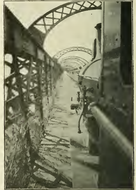
ORANGE RIVER BRIDGE, SOUTH AFRICA. BUSHES ON SIDE FACILITATE PASSAGE OF HORSES.
