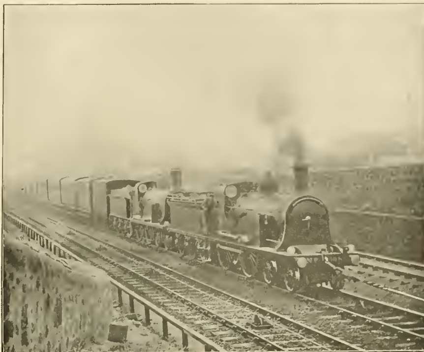
DOUBLE HEADER AND CABLE HELP ON COWLAIRS INCLINE.
