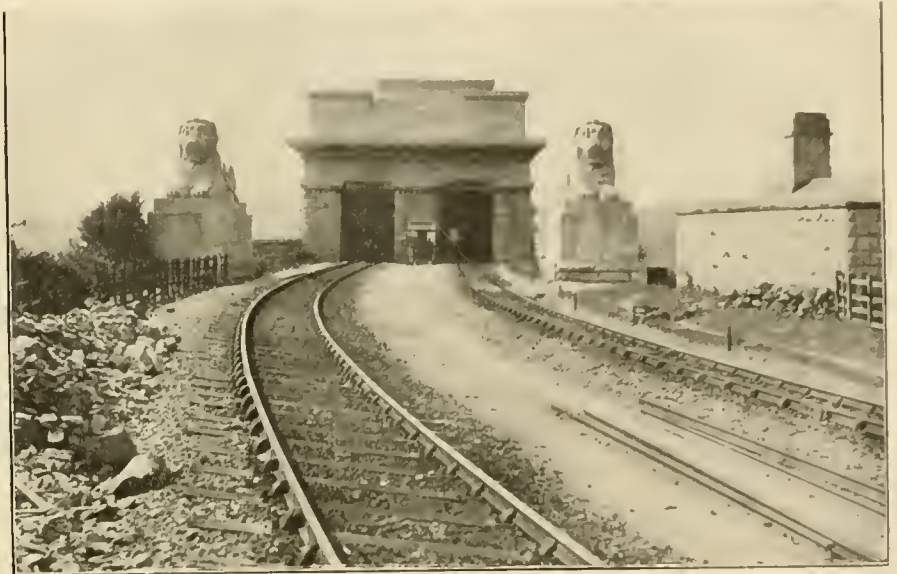
ENTRANCE TO THE BRITANNIA BRIDGE.
