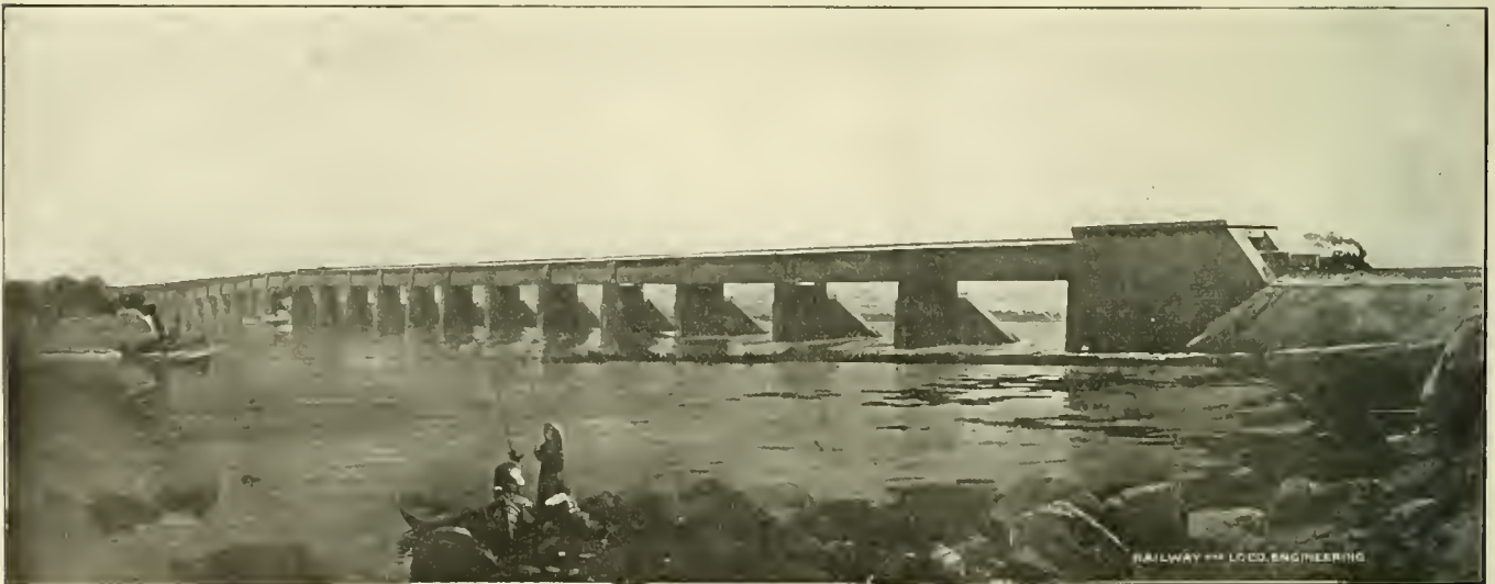
OLD VICTORIA TUBULAR BRIDGE OVER THE ST. LAWRENCE AT MONTREAL, CANADA.
