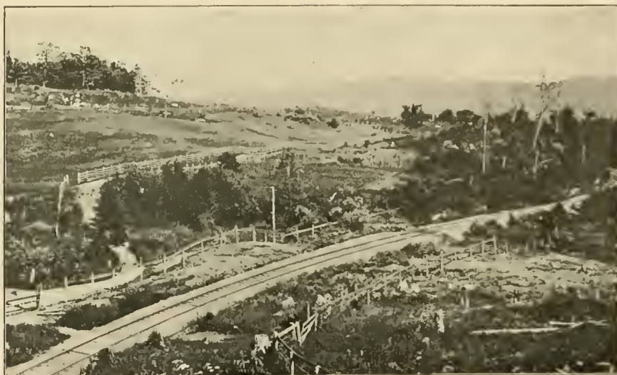
THE MODERN HIGHWAY OF COMMERCE.
