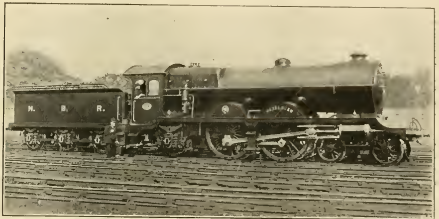
NORTH BRITISH 4-4-2 WITH BELPAIRE BOILER.
