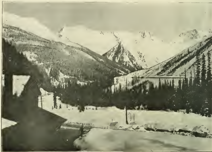
RAILROADING IN THE ROCKIES, WHERE THE ROTARY WORKS.
