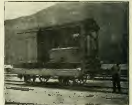
SAND BLAST CAR FOR RAIL BONDING.
