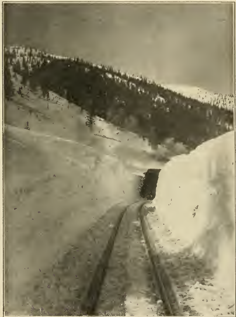
SNOW CUT BORED OUT BY THE ROTARY PLOW.
