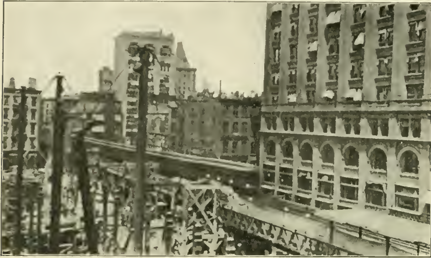
EXCAVATION IN NEW YORK FOR CORTLANDT STREET TERMINAL HUDSON COMPANIES' TUNNELS.
