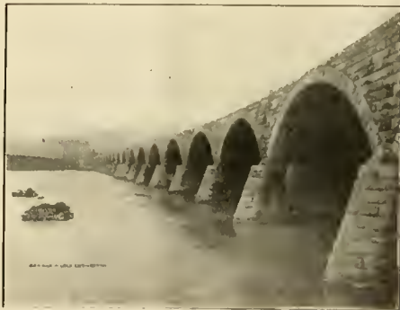
BRIDGE OVER THE SUSQUEHANNA RIVER AT ROCKVILLE, PA., ON THE PENNSYLVANIA.
