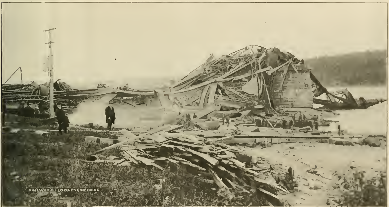
RUINS OF THE CANTILEVER BRIDGE OVER THE ST. LAWRENCE AT QUEBEC.
