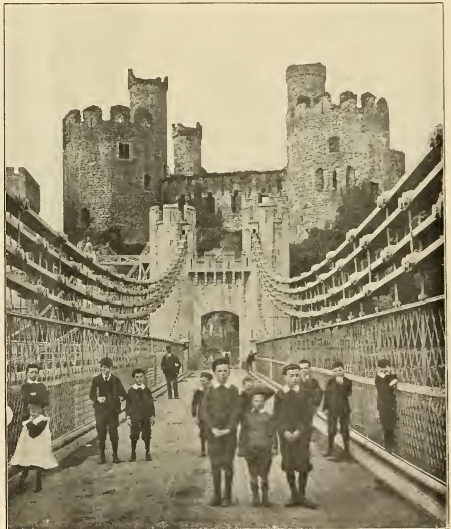
SUSPENSION BRIDGE AT CONWAY CASTLE, WALES, SHOWING EYE BAR SUSPENSION CHAINS.
