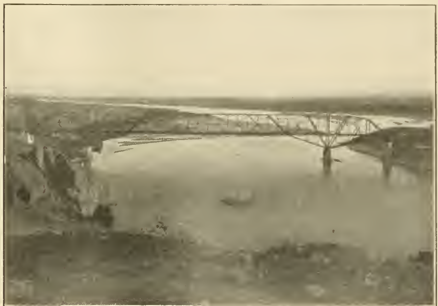
CANTILEVER BRIDGE ON THE A. T. & S. F., AT NEEDLES, CAL.
