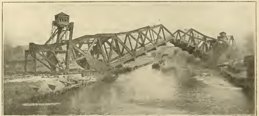
ROLLER LIFT BRIDGE. CHICAGO TERMINAL TRANSFER RAILROAD.
