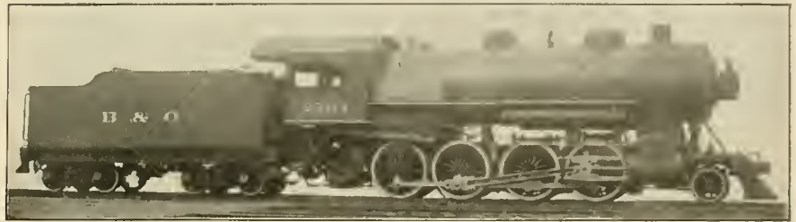
BALTIMORE & OHIO 2-8-0 ENGINE OF MODERN DESIGN.
