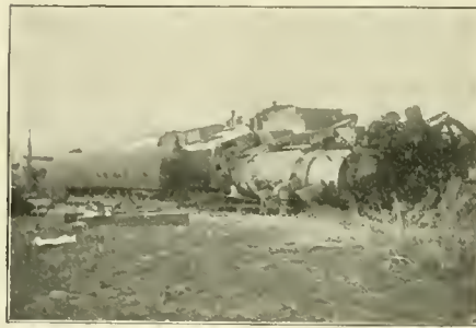
READY FOR THE WRECKING TRAIN.
