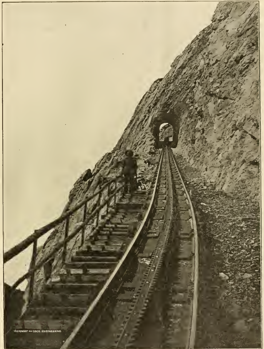
A BIT OF RACK AND PINION ROAD ON THE VERY EDGE OF THE ABYSS ALONG THE SHEER SIDE OF THE MOUNTAIN.
