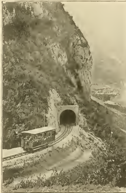
SALEVE ELECTRIC RAILWAY IN SWITZERLAND.
