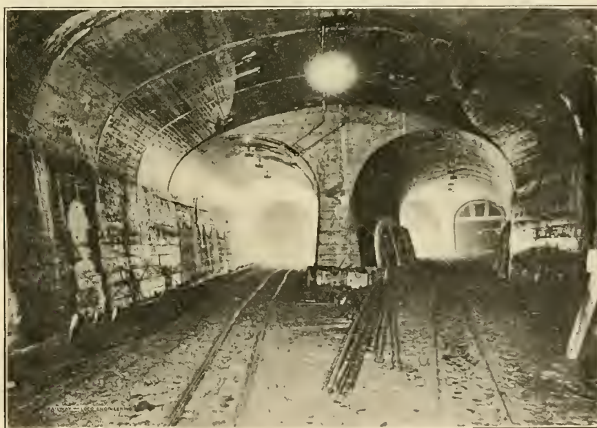
HUDSON COMPANIES' TUNNELS BELOW THE PENNSYLVANIA RAILROAD TERMINAL AT 34TH STREET, NEW YORK.
