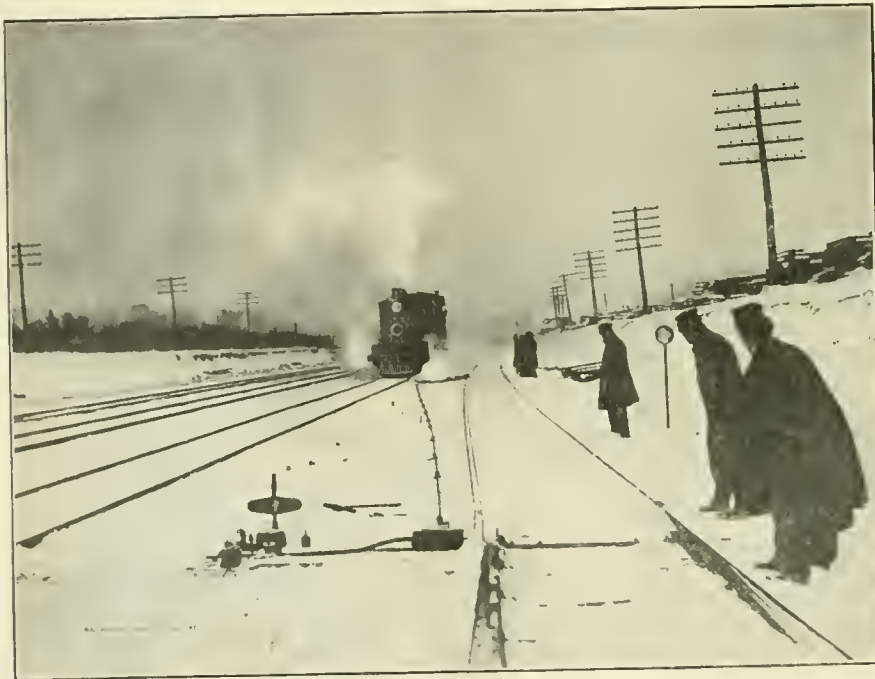
TESTING SWITCH CLOSING DEVICE ON THE L. S. & M. S. TRIP ON ONE TRACK CLOSES SWITCH ON ANOTHER TRACK, FOR EXPERIMENTAL PURPOSES.
