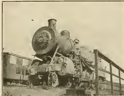
ON THE RAILS AGAIN.
