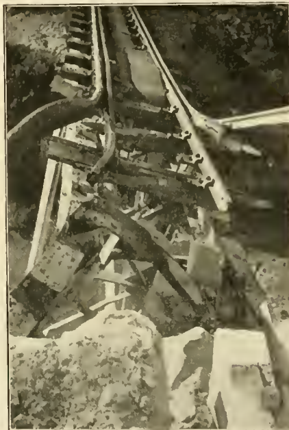
TWISTED PORTION OF SECOND SPAN OF AVOCA BRIDGE, SOUTH AFRICA.
