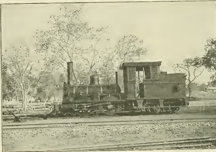
ENGINE ON THE RAJAPUKANA MALWA RAILWAY, INDIA.
