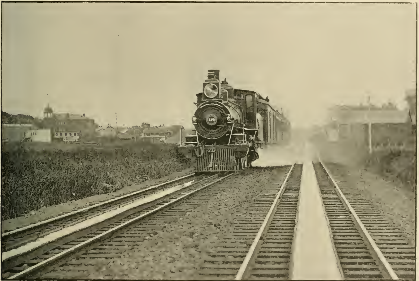
TRACK TANKS ON THE N. Y. & L. B., NEAR LONG BRANCH, N. J. ENGINE SCOOPING UP WATER.
