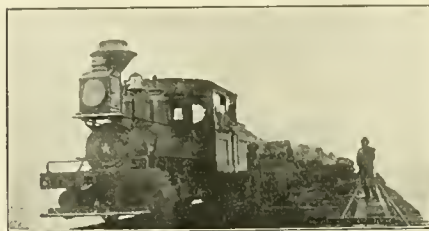
ROCK TRAIN, COLUMBIA RIVER JETTY.
