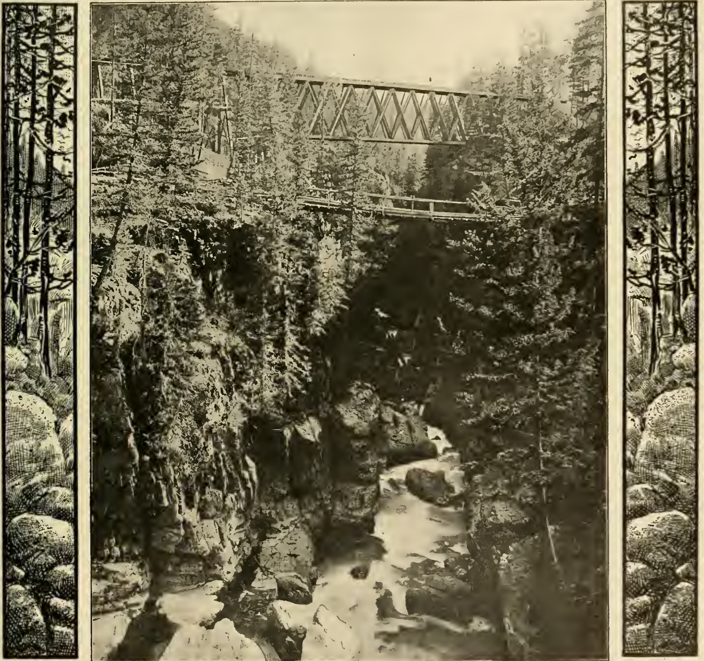
HOWE TRUSS RAILWAY BRIDGE AND LIGHT CARRIAGE ROAD BRIDGE CROSSING A DEEP MOUNTAIN GORGE.
