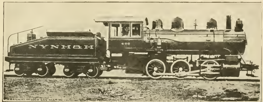
SWITCHING "PUG" ON THE NEW HAVEN.
