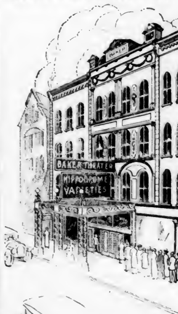
The Baker Hipp Building, of Varieties, in Rochester, N. Y., after being remodelled and refitted, reopened with vaudeville on October 23, under the management of Elmer J. Walters, who also manages Greater Ontario Beach Park at Rochester during the summer. A ten-piece singing orchestra is one of the novelties. Nine acts are used each week.
