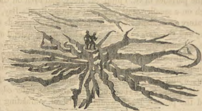
Fig. 4.—Fissures near Jerocarne in Calabria, raised by the earthquake of 1783.
