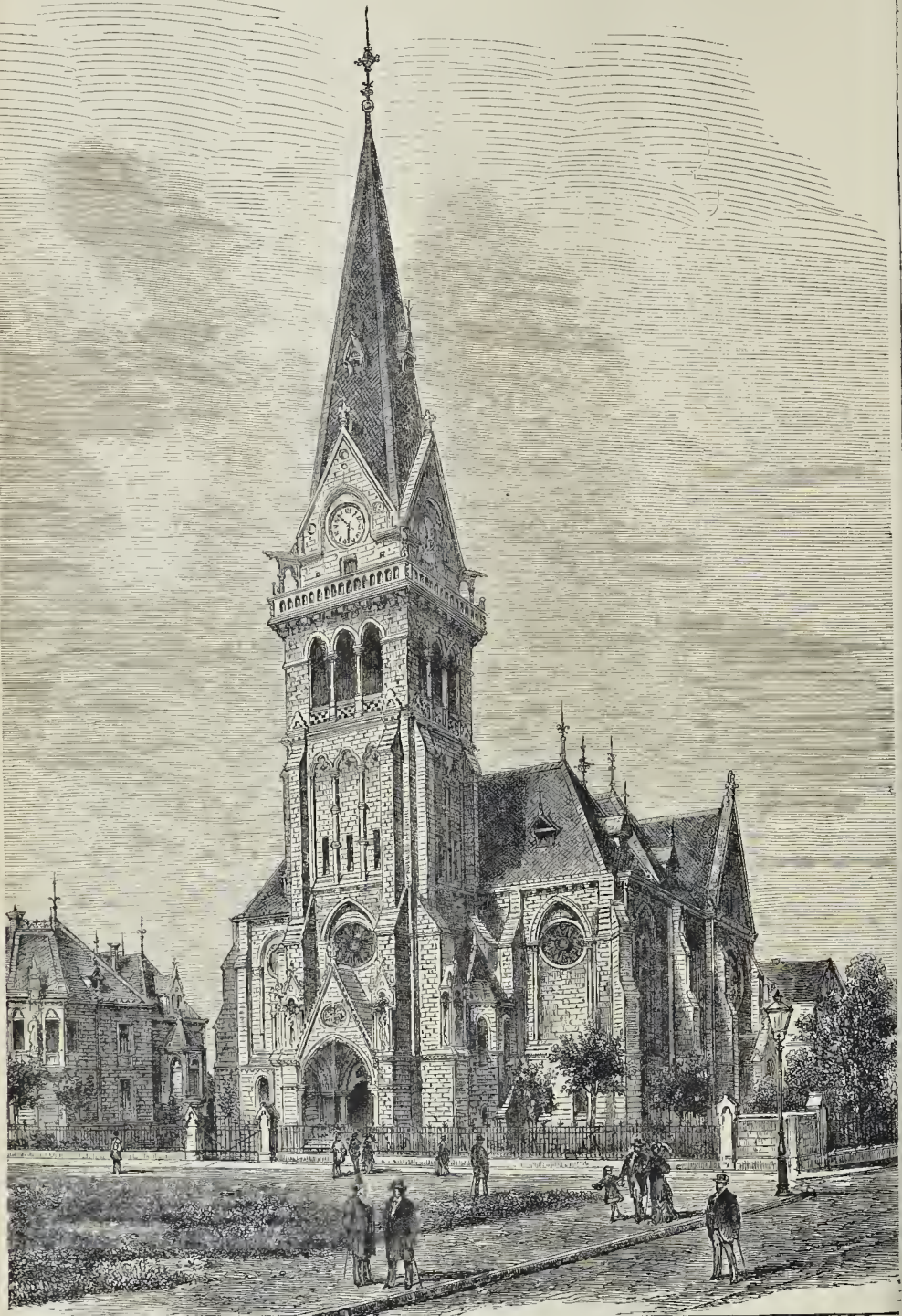
ST. SAVIOUR'S CHURCH, STRIESEN, DRESDEN.—HERR G. L. MÜCKEL, DRESDEN, ARCHITECT.
