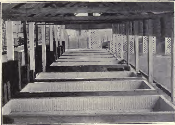
A "BATTERY" OF SHEETING TANKS (PATALLING ESTATE). DILUTION TANKS, RAISED, ON THE LEFT.
