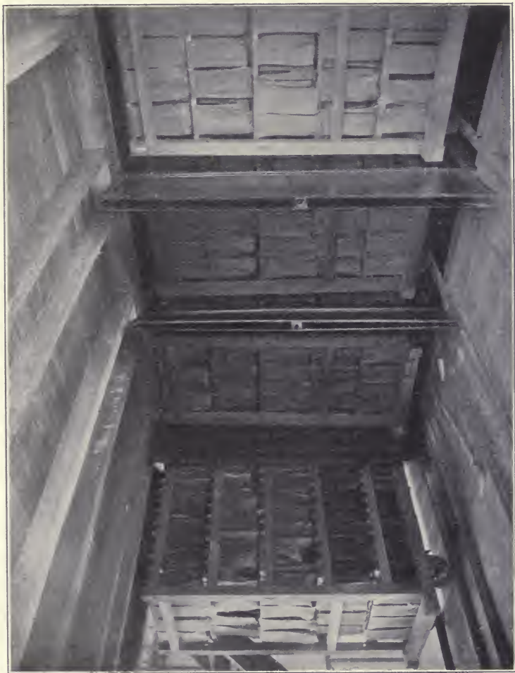
VIEW OF PLATFORM OF "DEVON" SMOKE-HOUSE; DOORS OF COMPARTMENTS OPEN, AND ONE RACK PARTIALLY WITHDRAWN.
