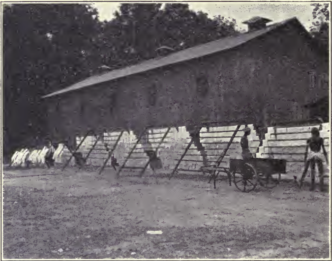
LARGE SMOKE-HOUSE OF ORDINARY CONSTRUCTION, WITH SHIELDED VENTILATORS PERMANENTLY OPEN.
