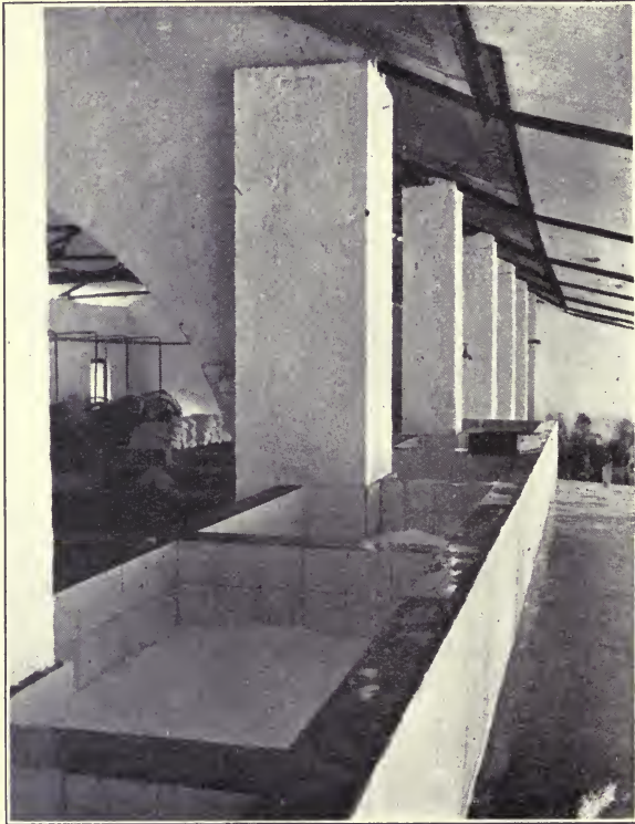
ANOTHER SET OF DILUTION TANKS ON RAISED VERANDAH.
